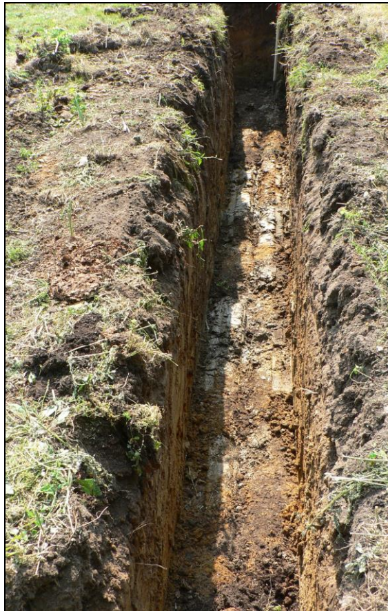
Southern trench of garage
