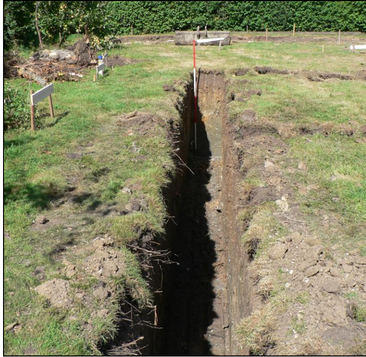
Western trench for house from south
