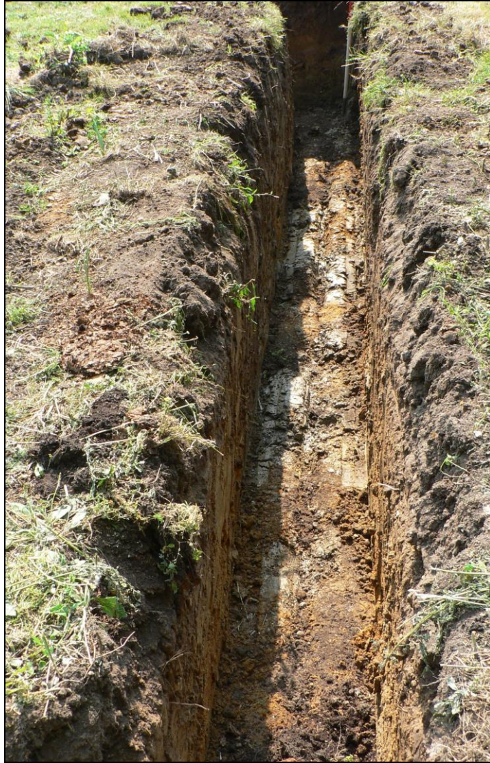
Southern trench for new house
