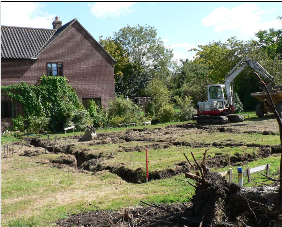
New house area from northwest
