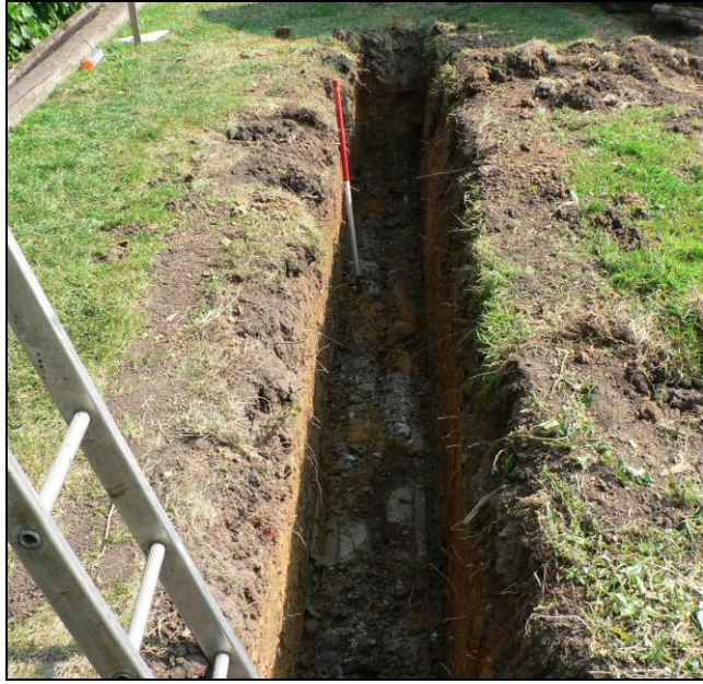
Northern trench of garage
