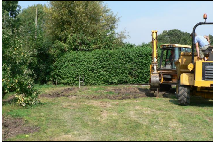
General view of garage area from south
