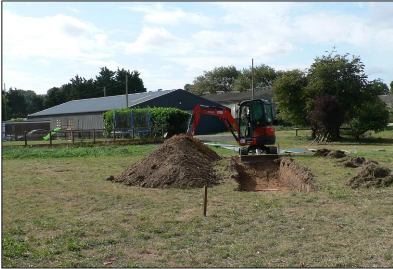
General view from southwest
