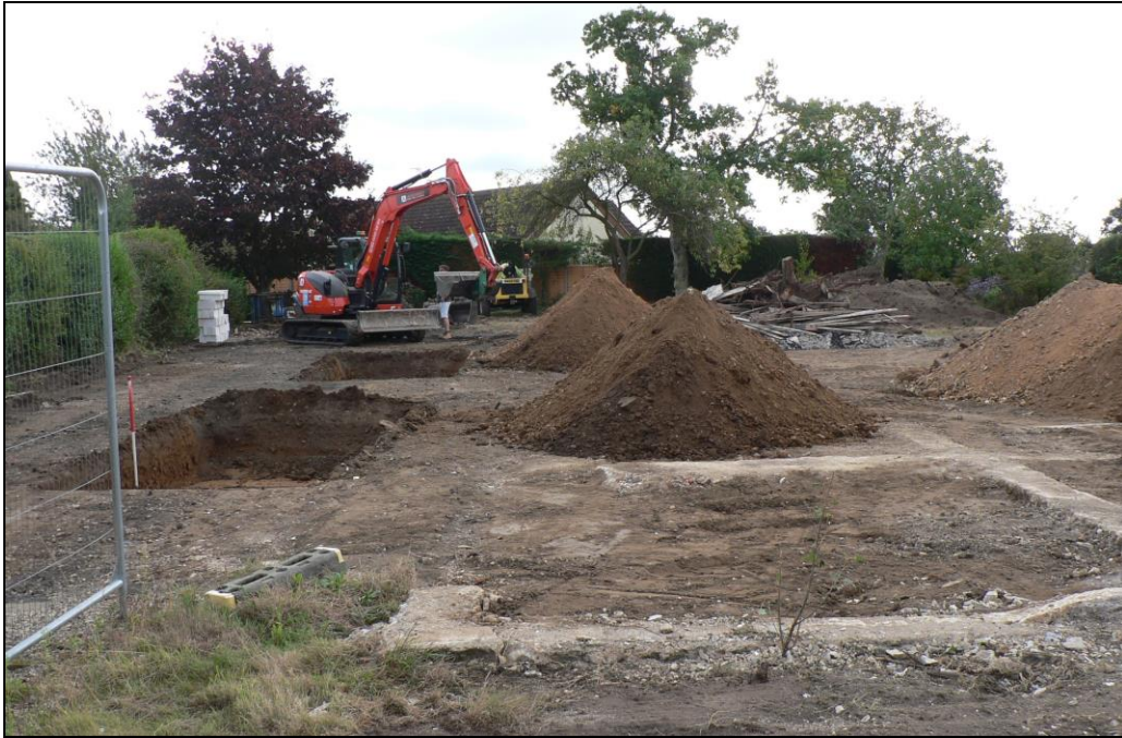
General view from west
