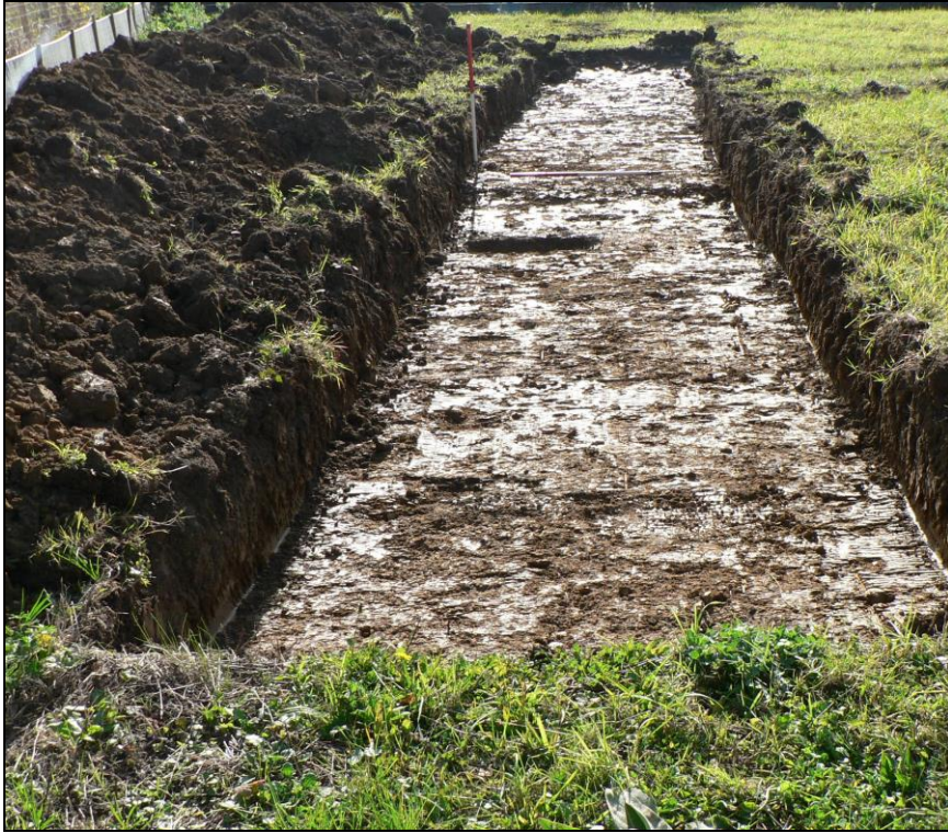
Trench 9 from northwest
