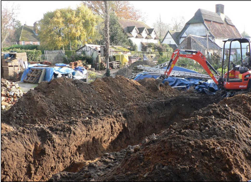
General view from northwest with Forge Cottage in background
