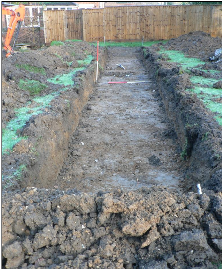
Trench 5 from south
