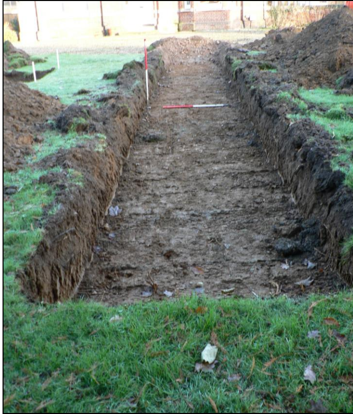
Trench 7 from south
