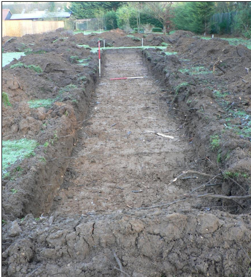
Trench 3 from south
