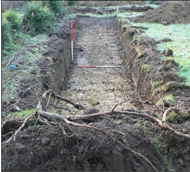
Trench 9 from north
