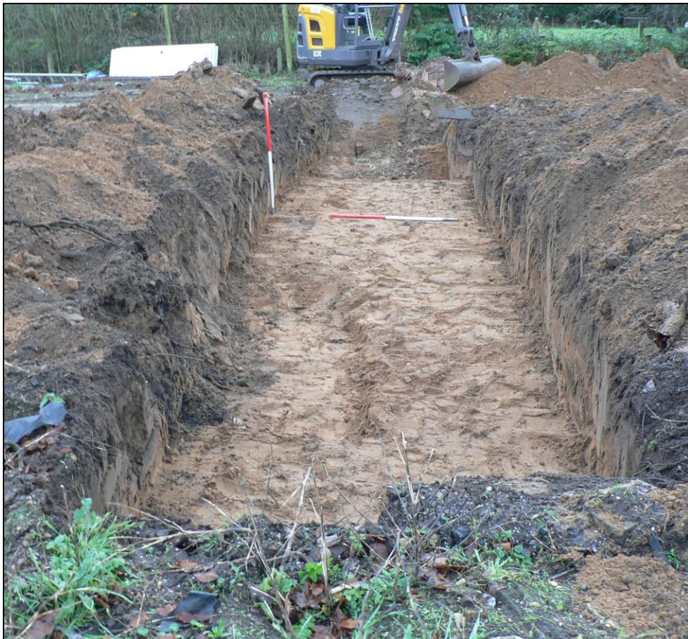
Trench 1 from west
