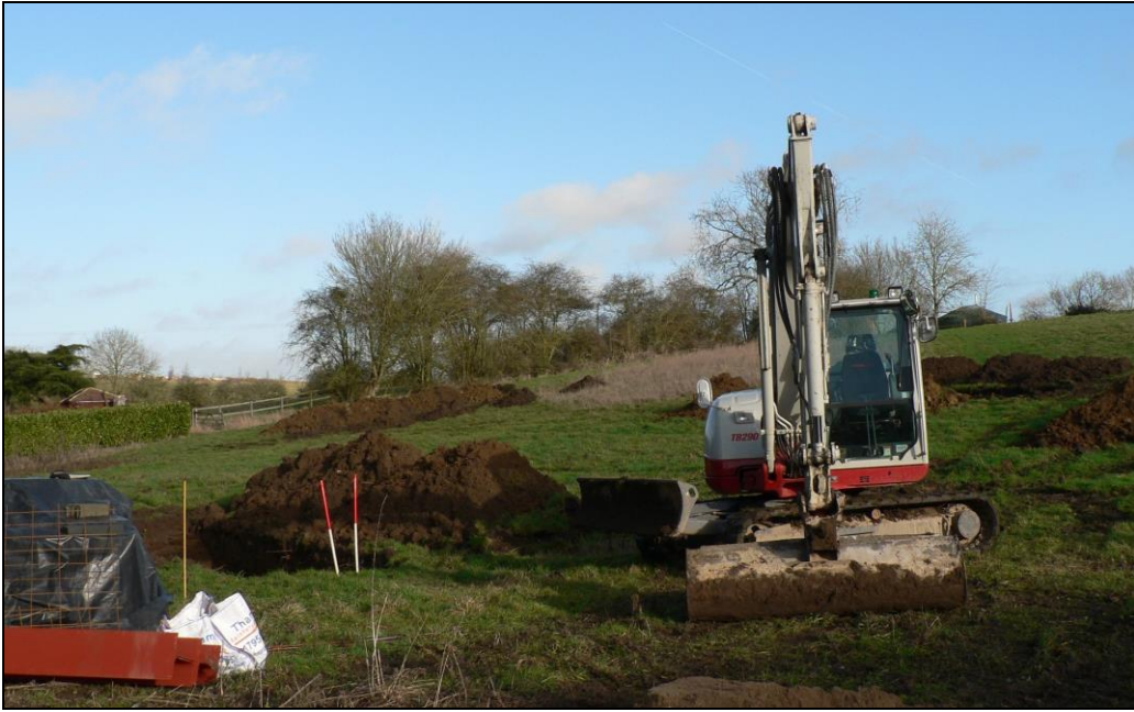
General view from southwest
