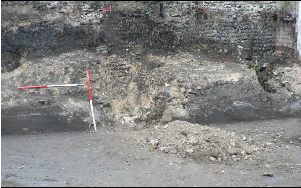
P3 Western wall from east
