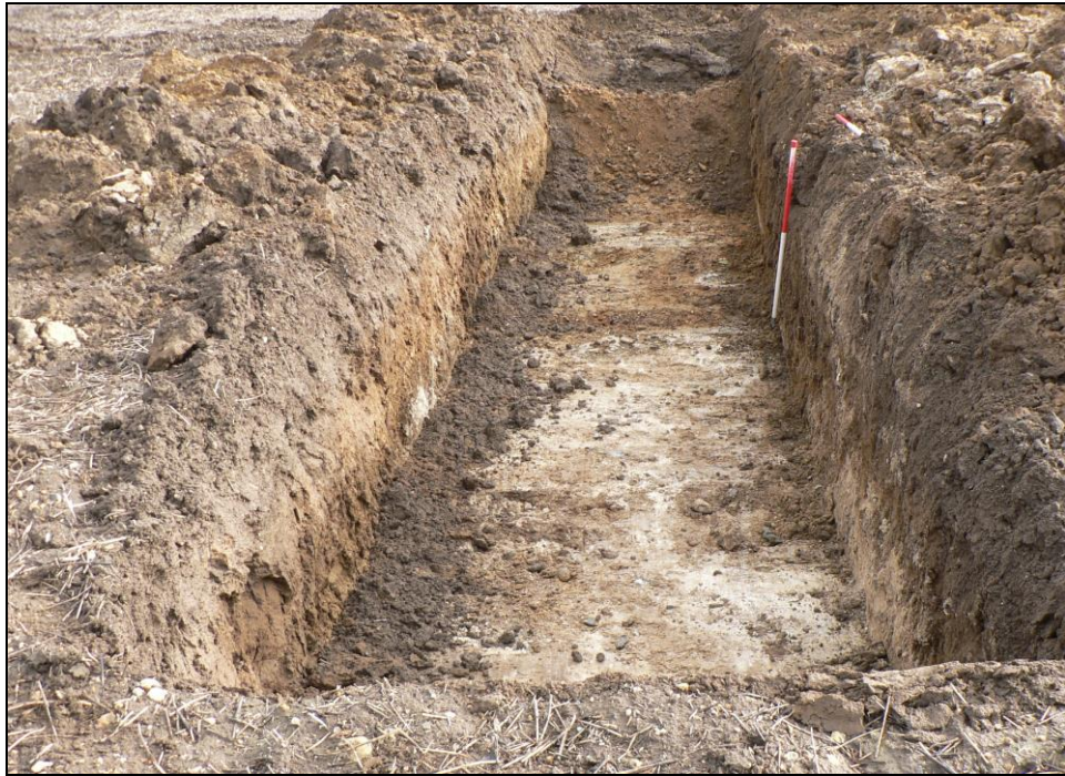
Trench 4 from north
