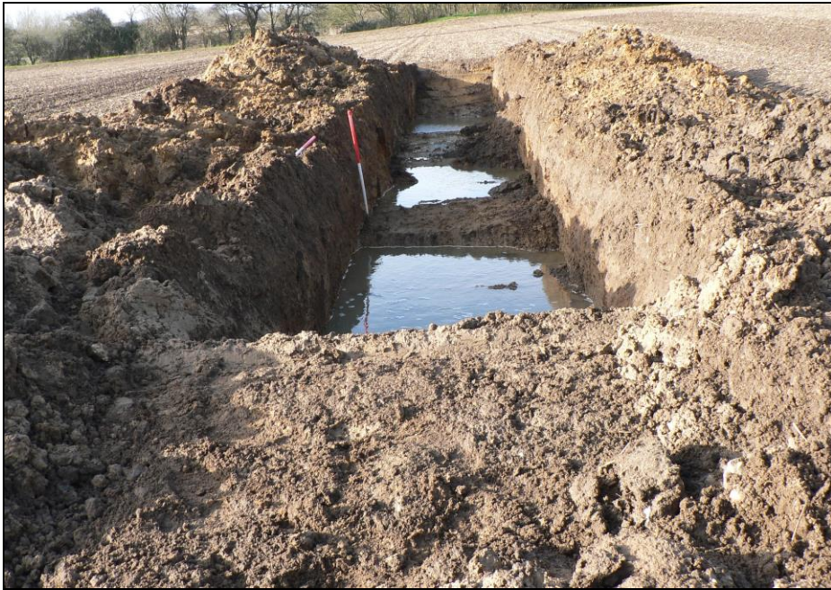
Trench 2 from east
