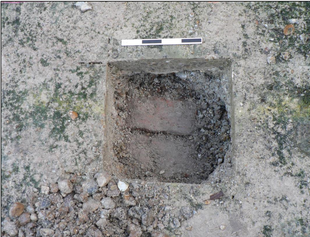
Brick foundation in pit 1
