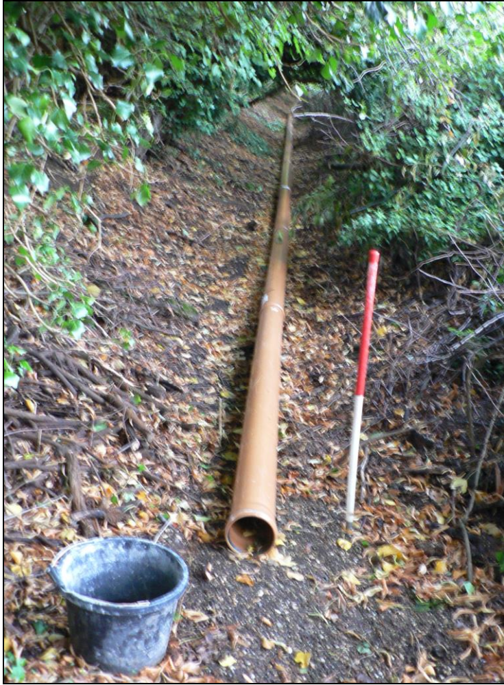
Drainage pipe in ditch
