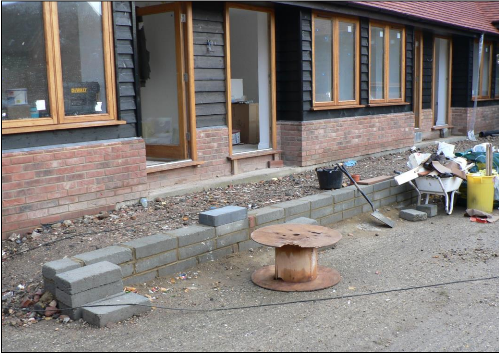
New accommodation blocks on concrete yard
