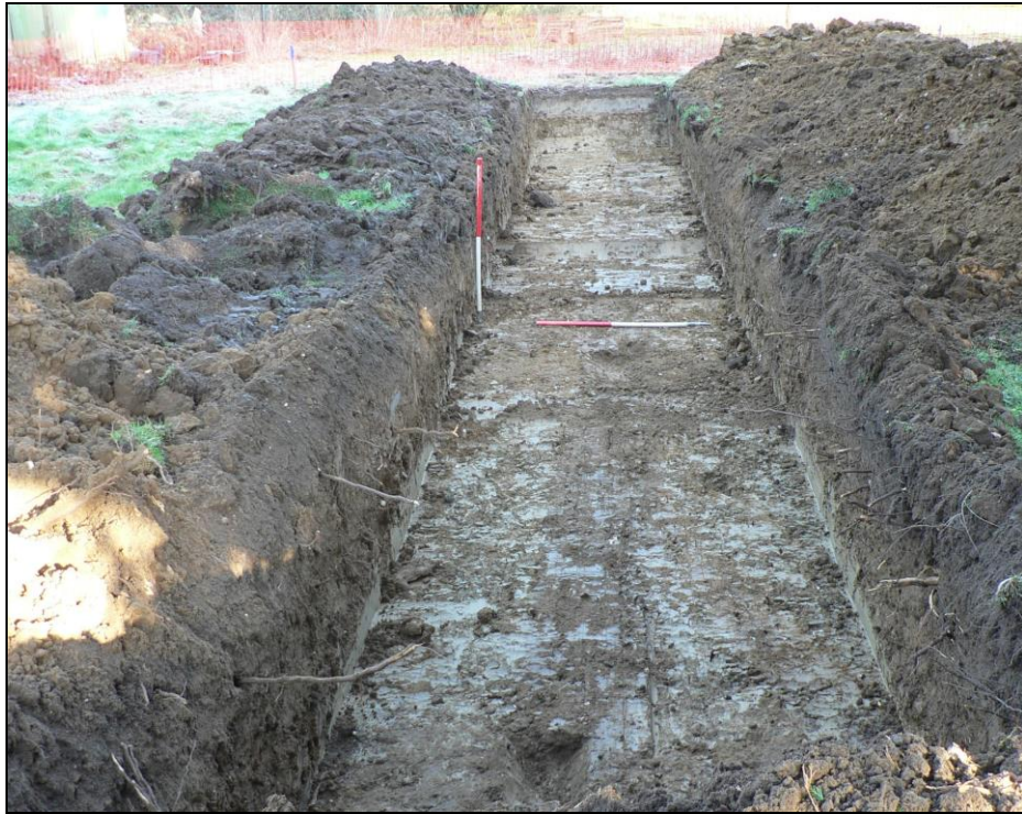
Trench 1 from south
