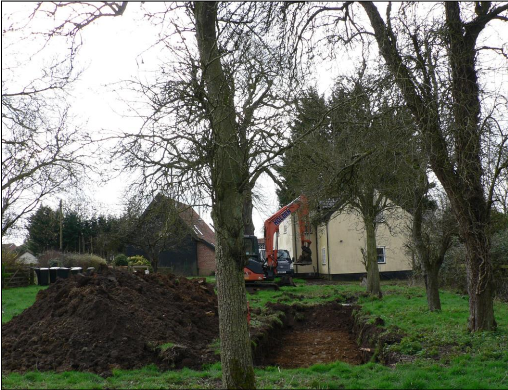
General view from north
