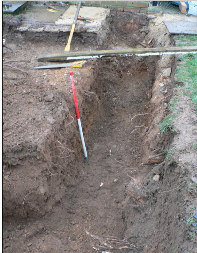
Western trench from north
