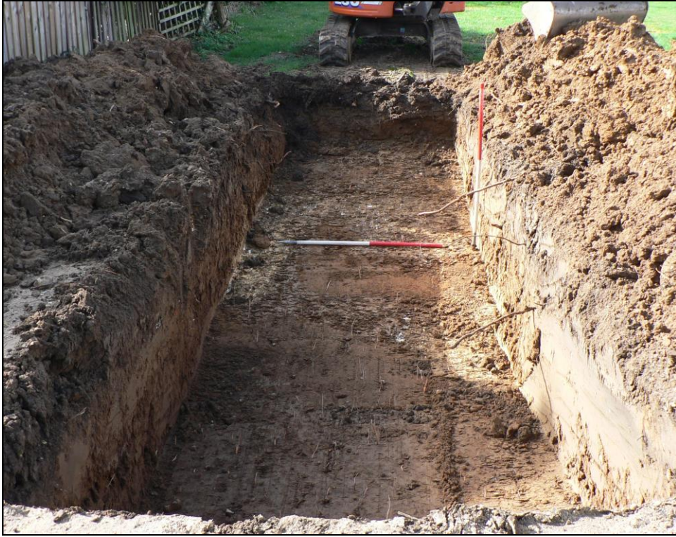
Trench 2 from northeast
