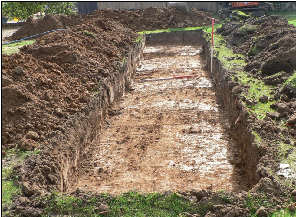
Trench 1 from northwest
