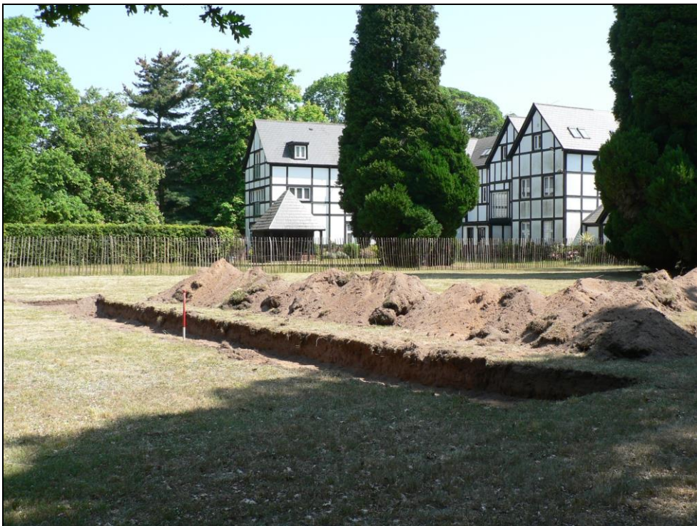
General view from northwest
