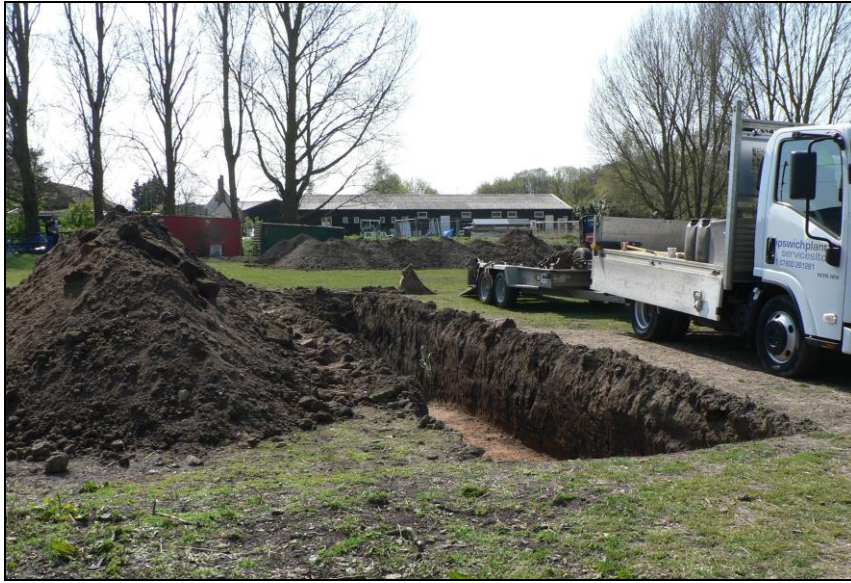
General view from north
