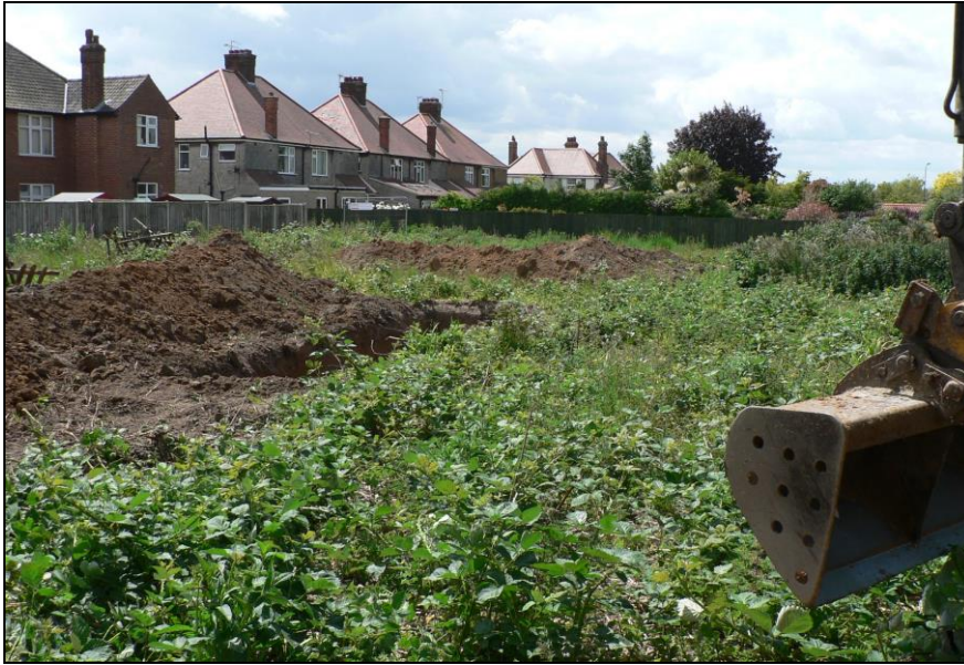
General view from northeast
