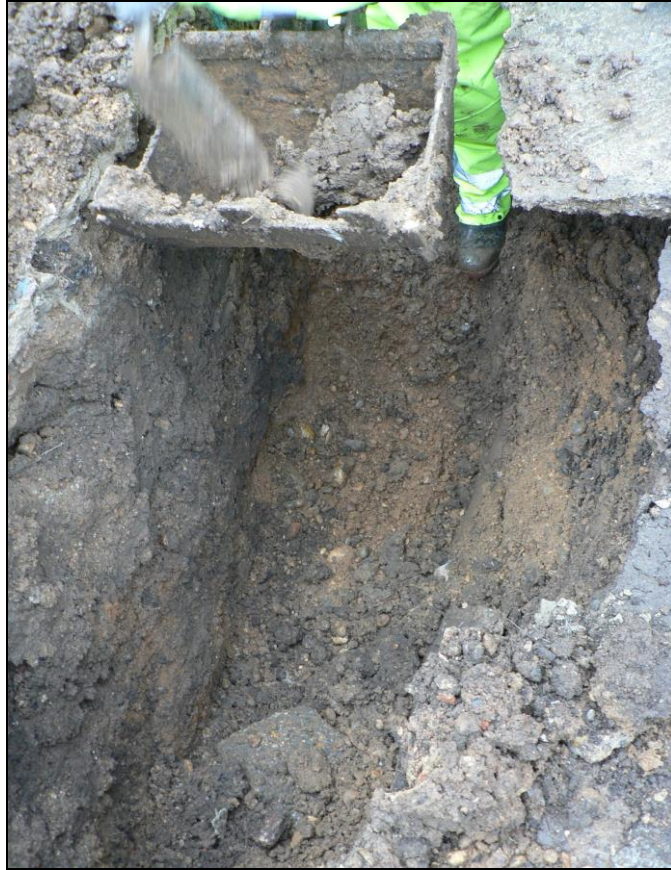
Rear extension trench
