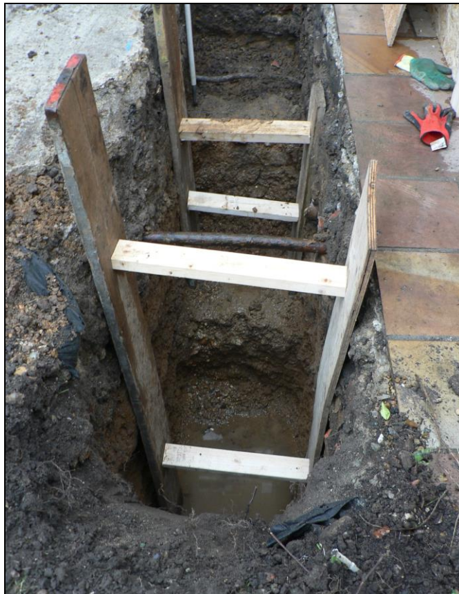
Rear extension trench
