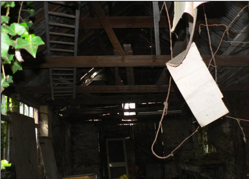
Interior of cart lodge building
