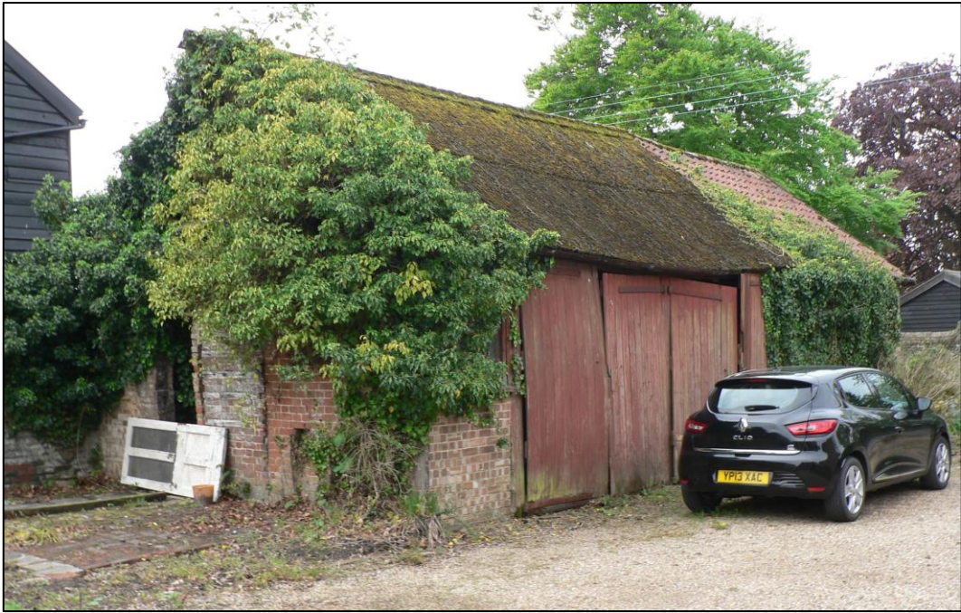
Cart lodge building from northeast
