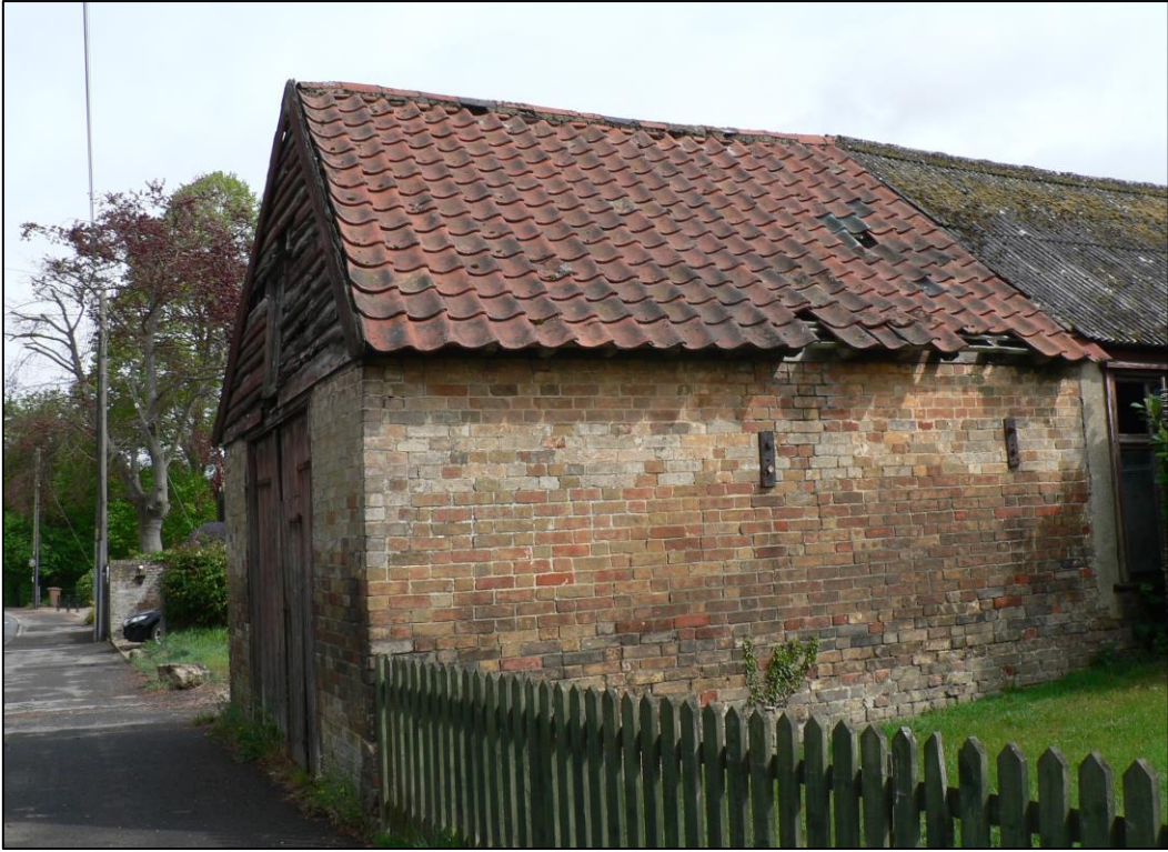
Cart lodge outbuilding from front
