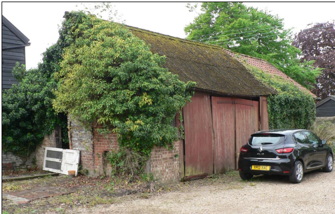
Cart lodge building for conversion from northeast
