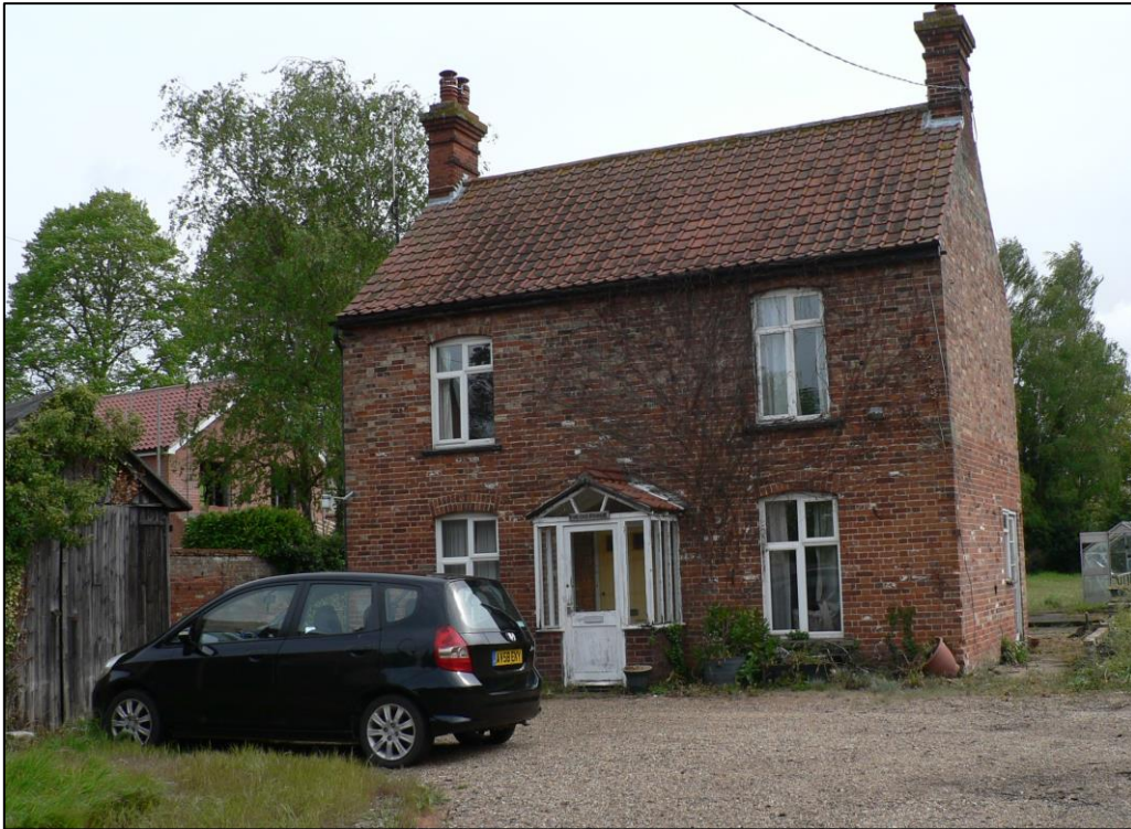
The Old Forge from west
