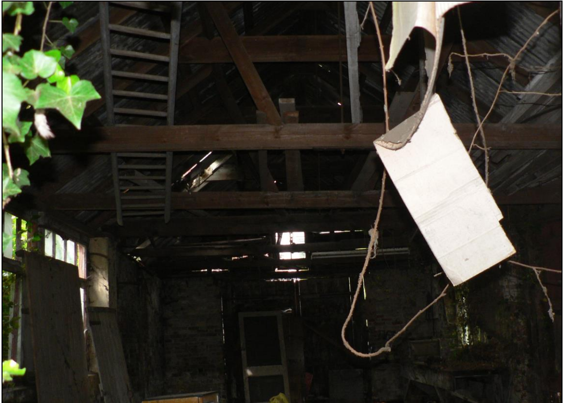
Interior of cart lodge building
