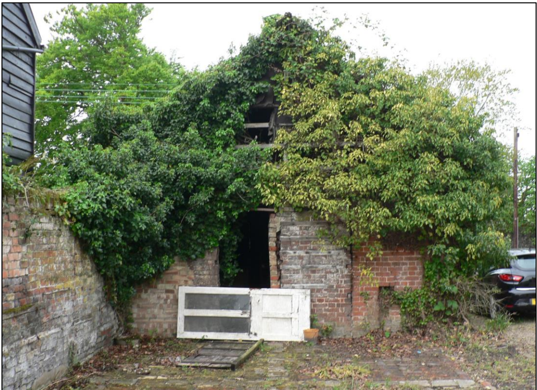
Cart lodge building from east
