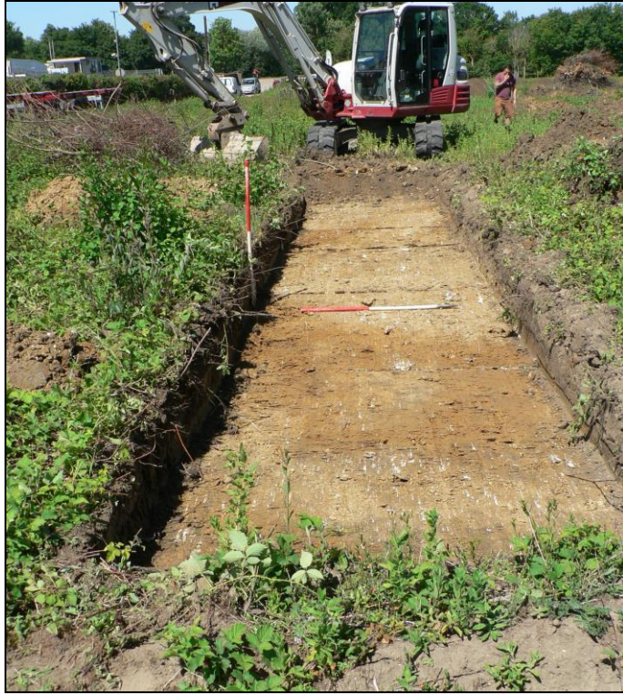
Trench 1 from east (western part)
