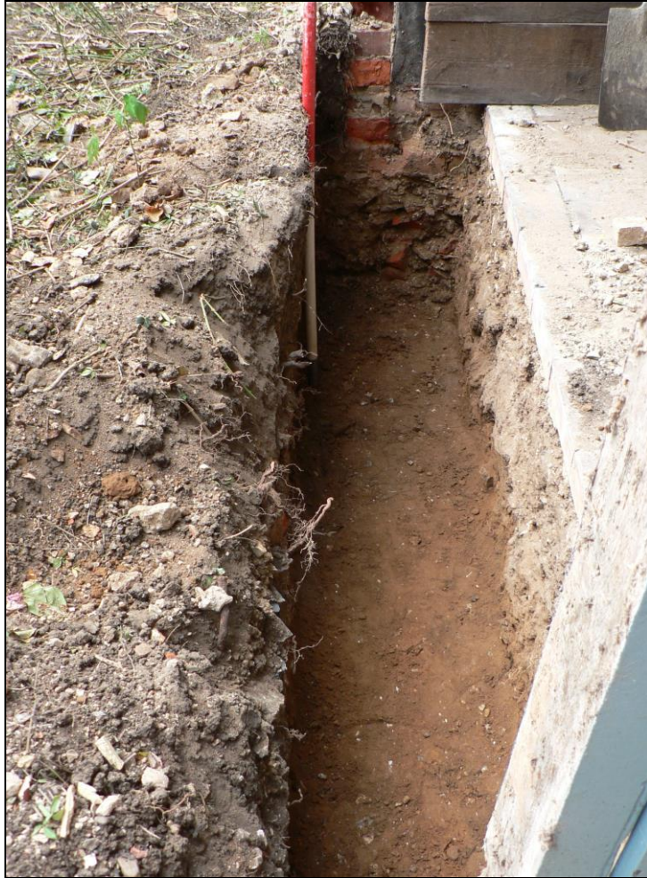
Eastern foundation for rear extension at full depth
