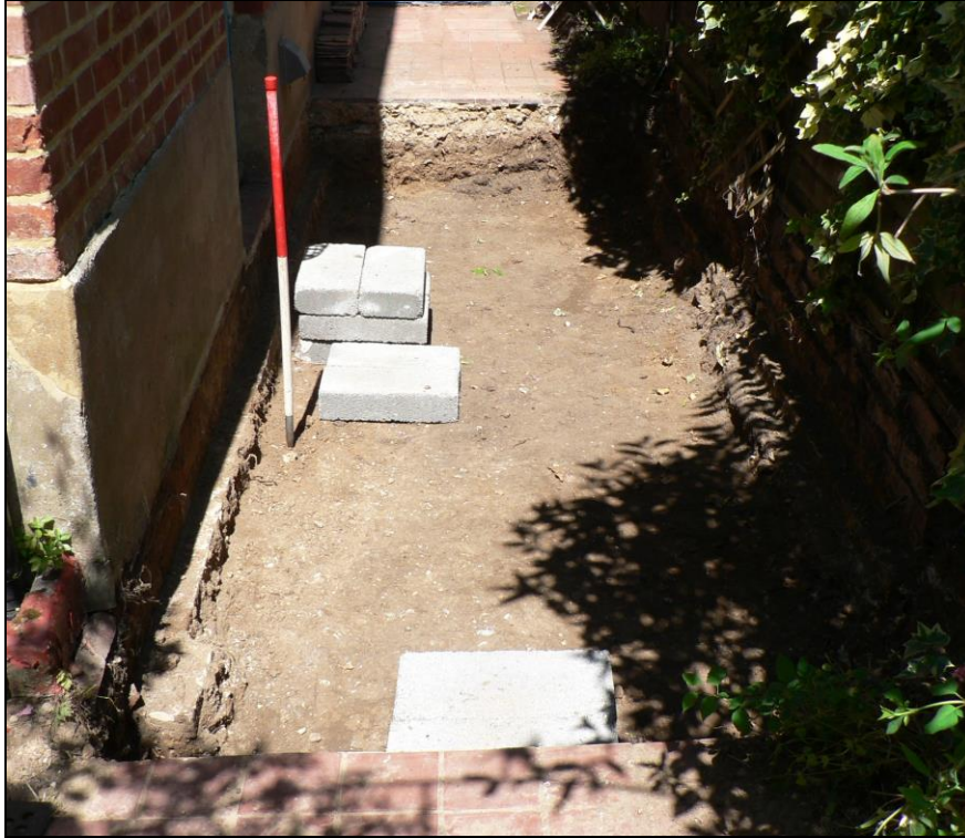
Initial excavation of side extension area to depth of 500mm
