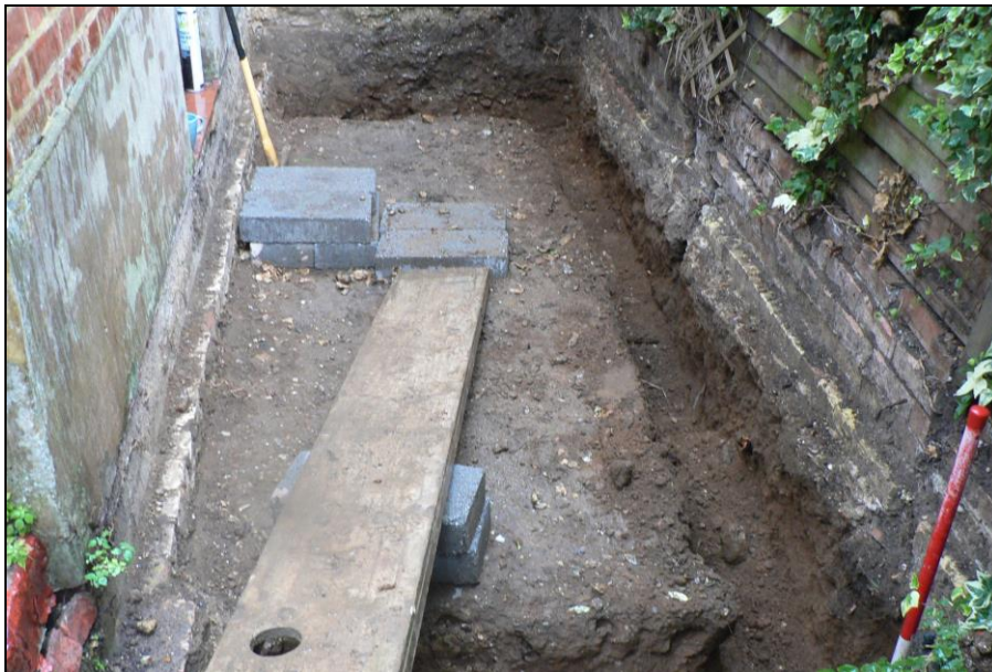
Excavated trenches for side extension at full depth
