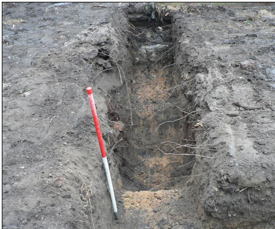
Western trench of main foundation trench with soakaway pit
