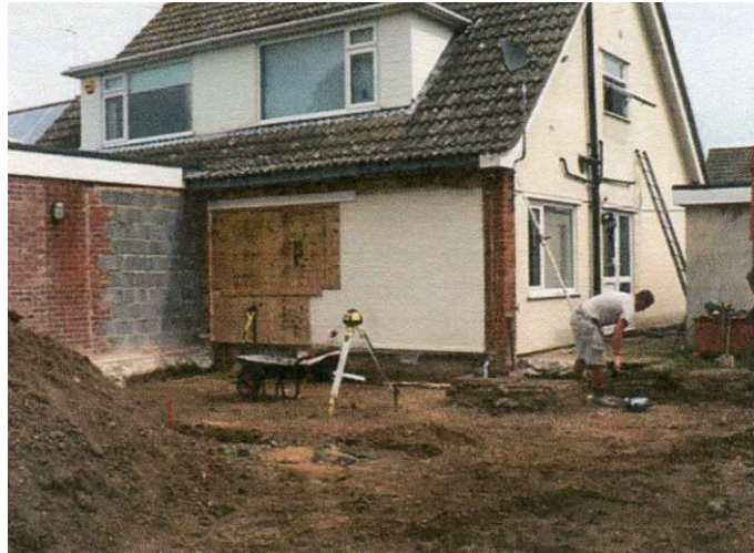
General view from southwest
