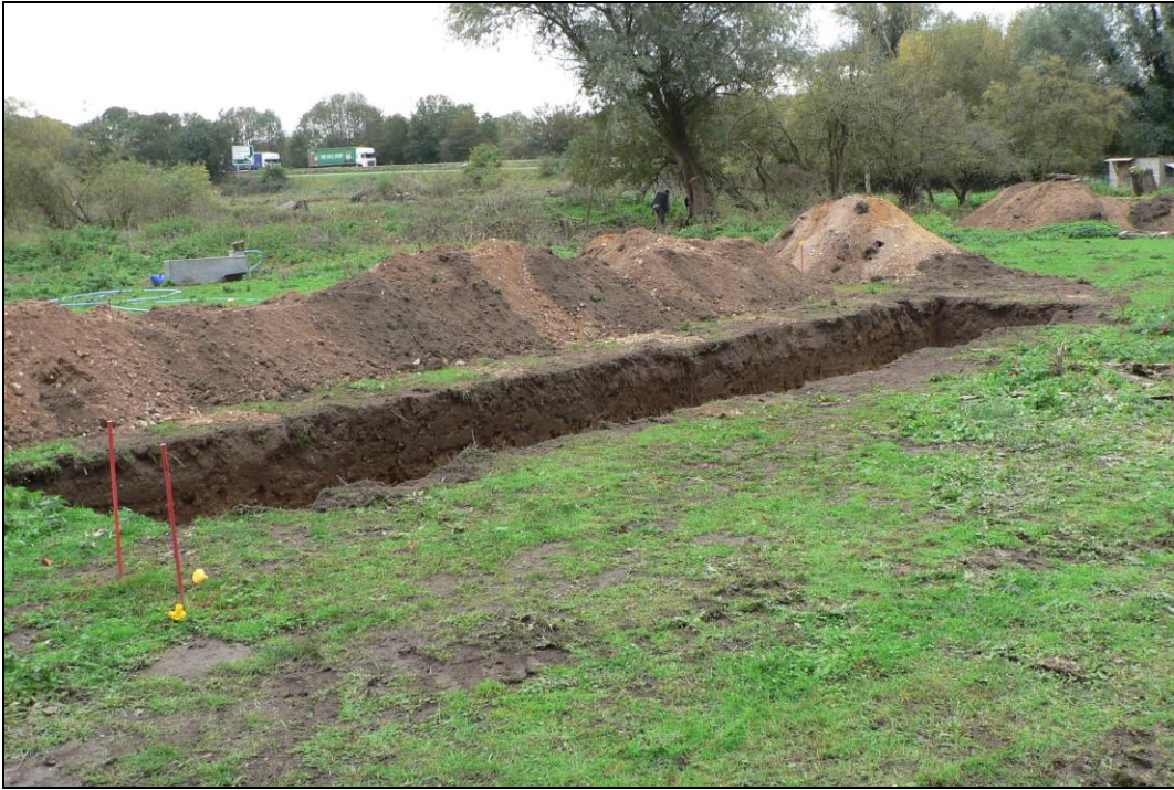
General view from northeast
