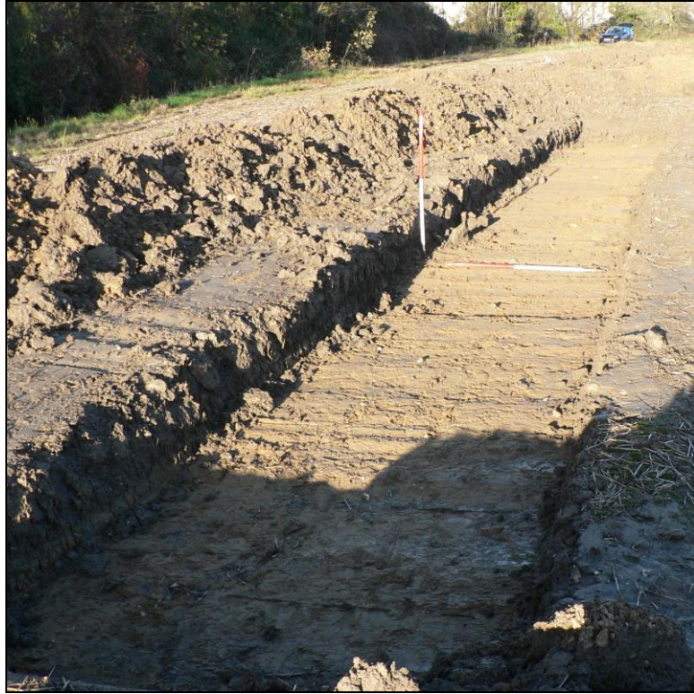
Trench 3 from south
