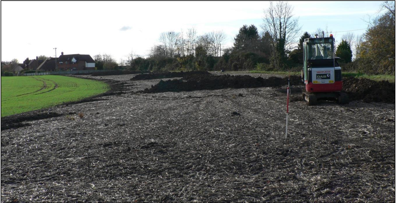
General view from north
