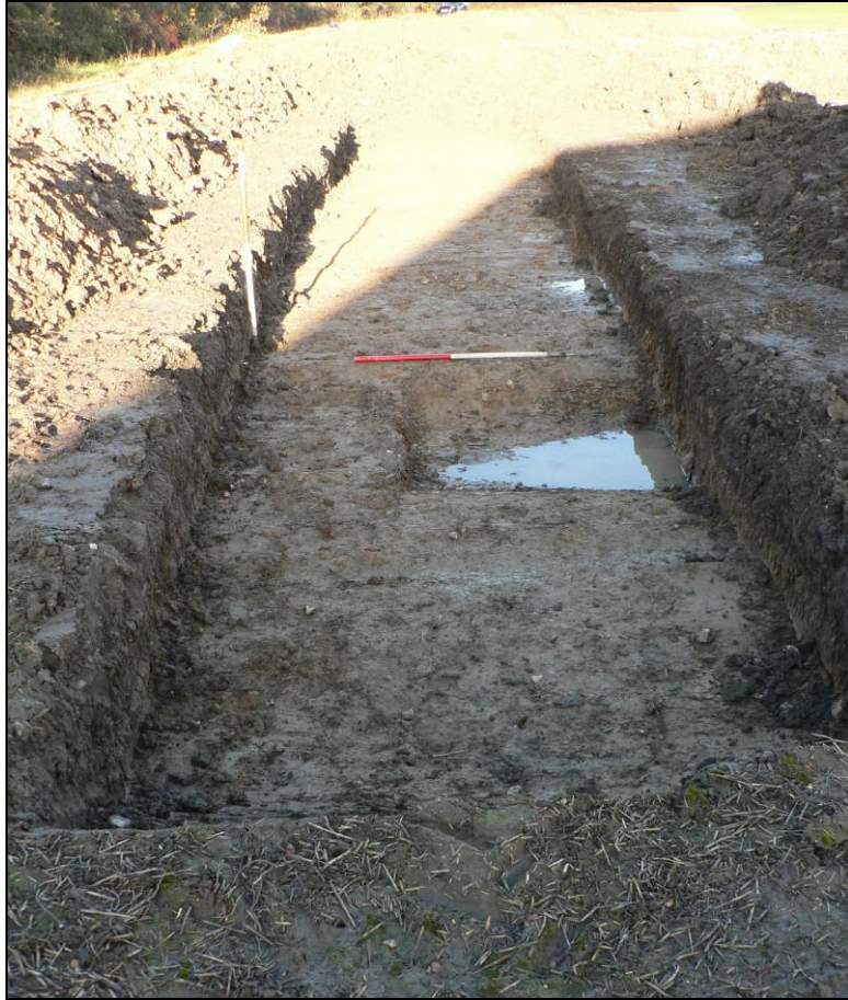
Trench 1 from north
