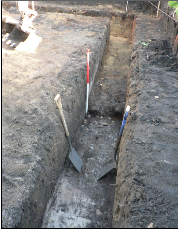
Southern foundation from east
