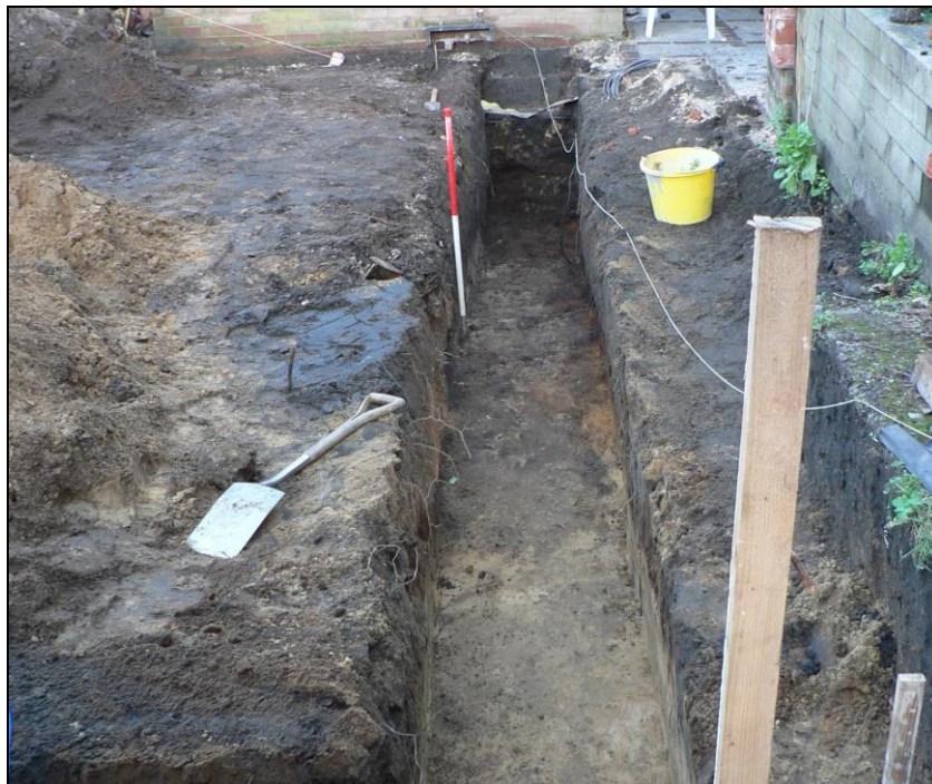
Western foundation from south
