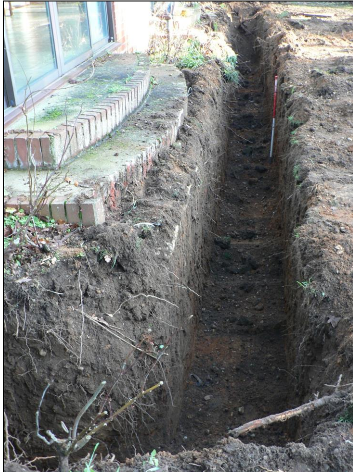
Rear extension trench from west
