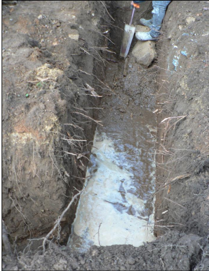
Southern end of side extension trench
