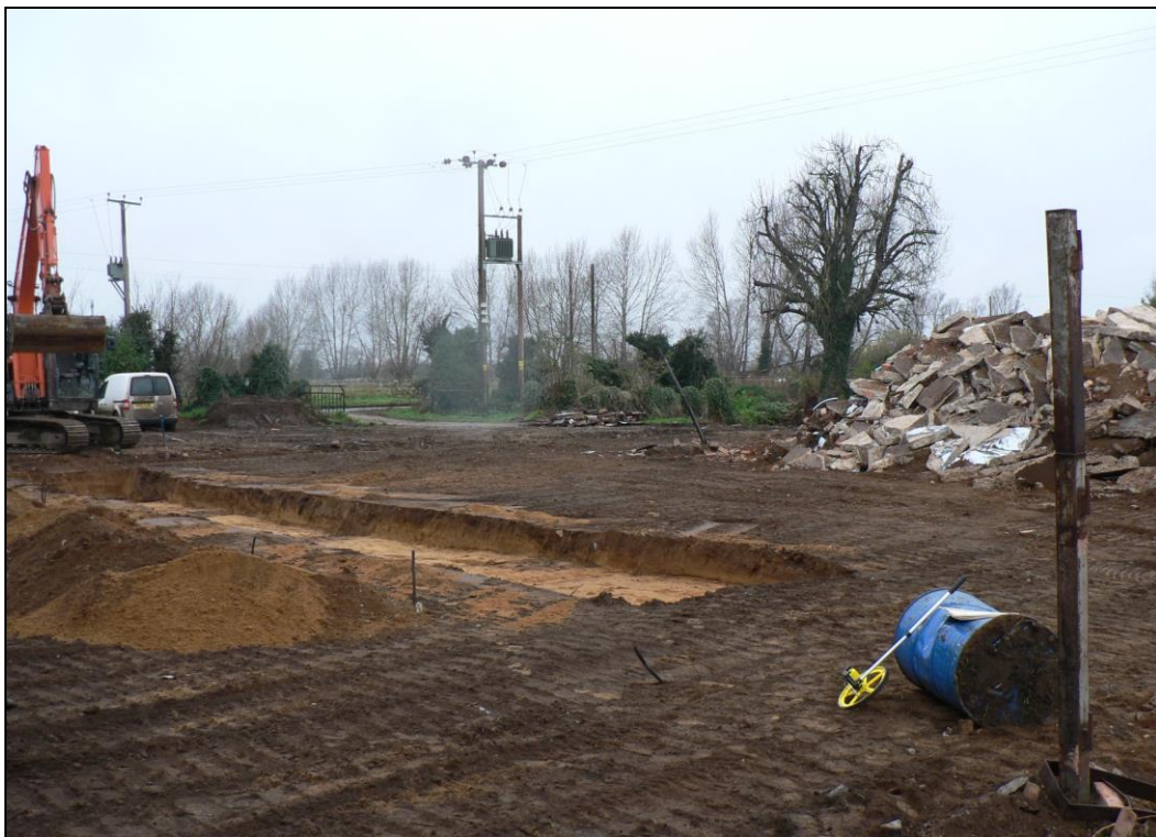
General view from southeast
