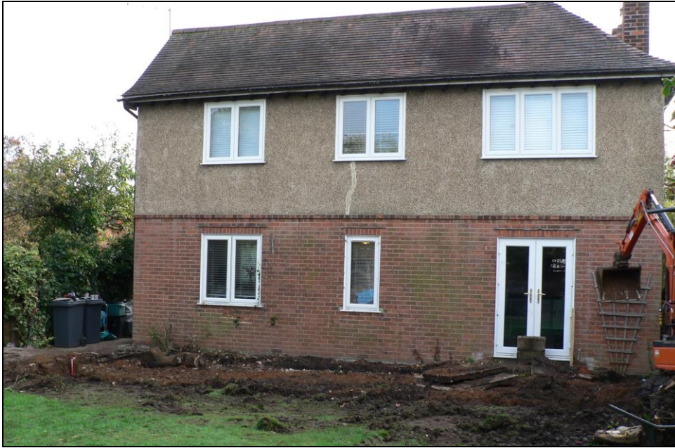
General view from west
