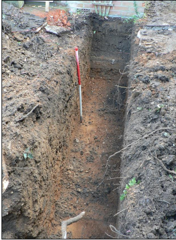
Southern trench from west
