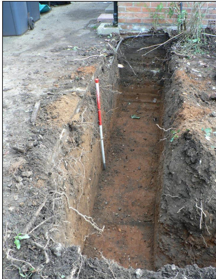
Northern foundation from west
