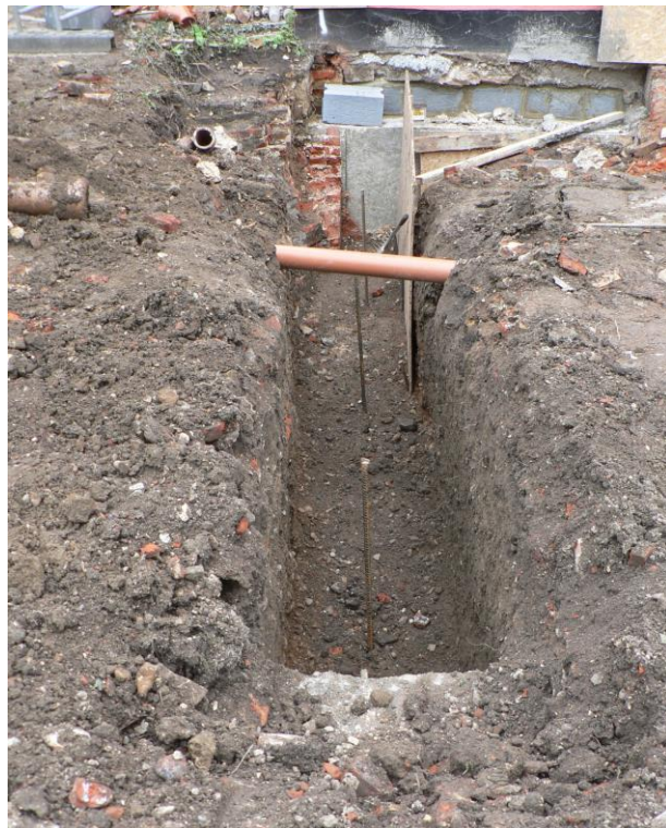
Eastern foundation trench from south
