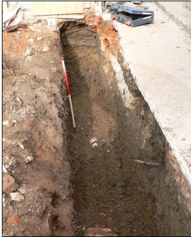
Western foundation trench from south
