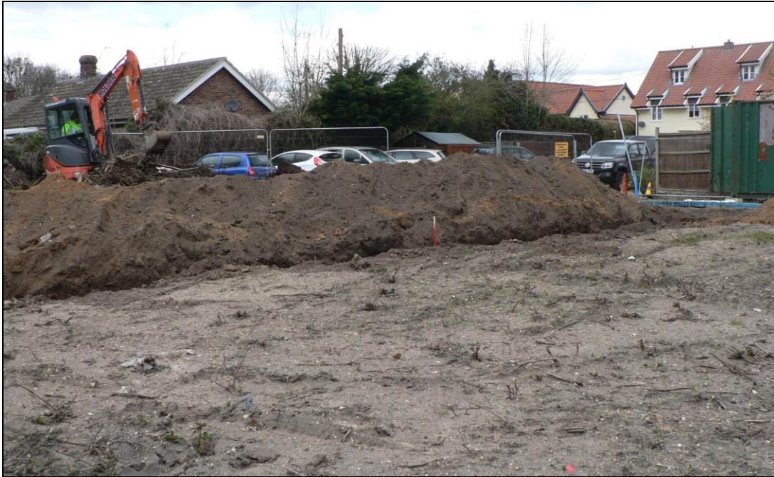
General view from southeast
