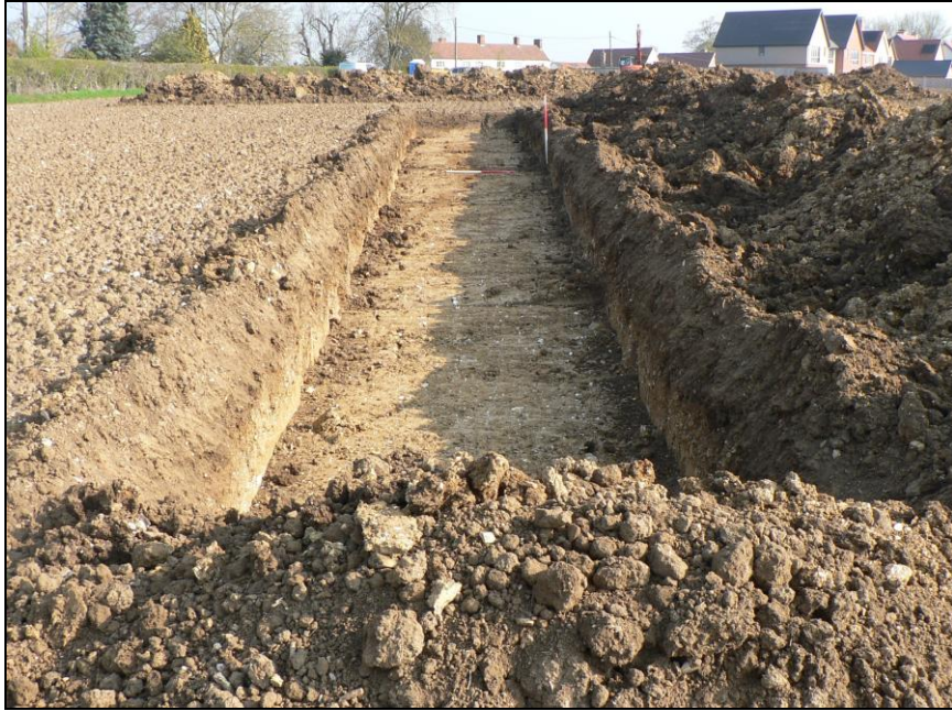
Trench 6 from south
