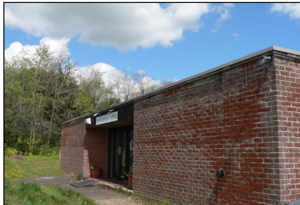
West side of community centre
