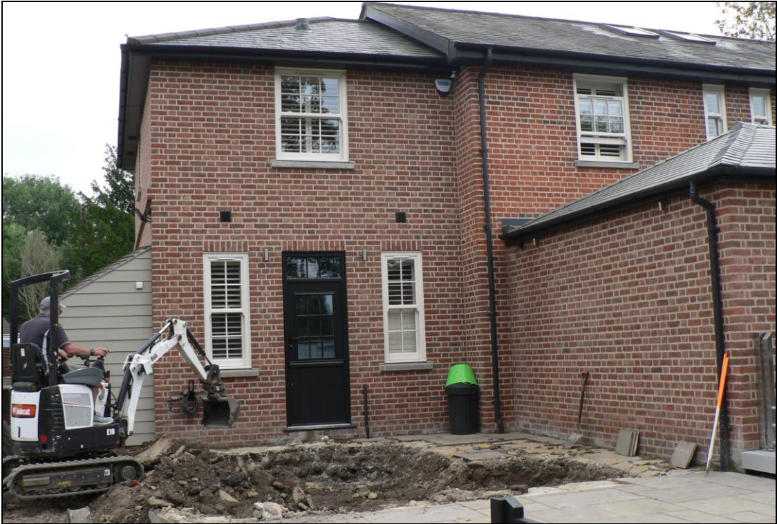
General view from north
