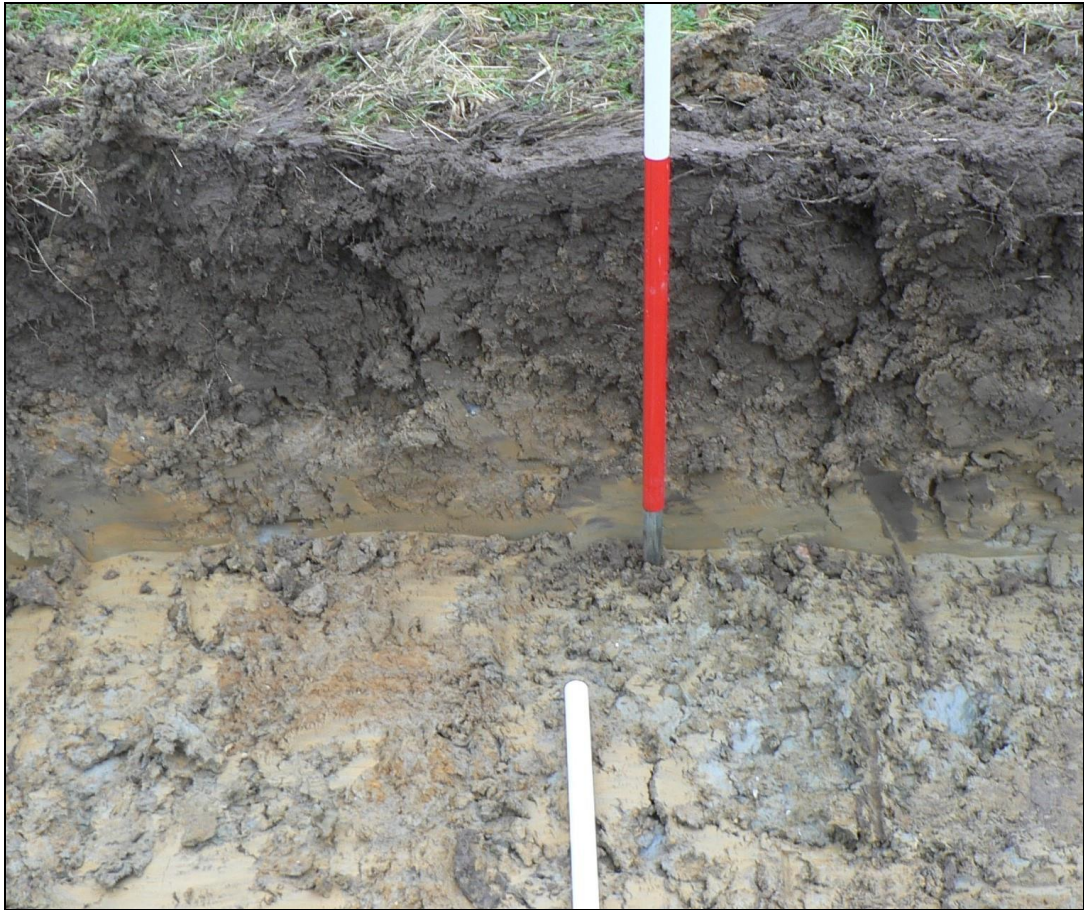
Trench 4 deposit profile
