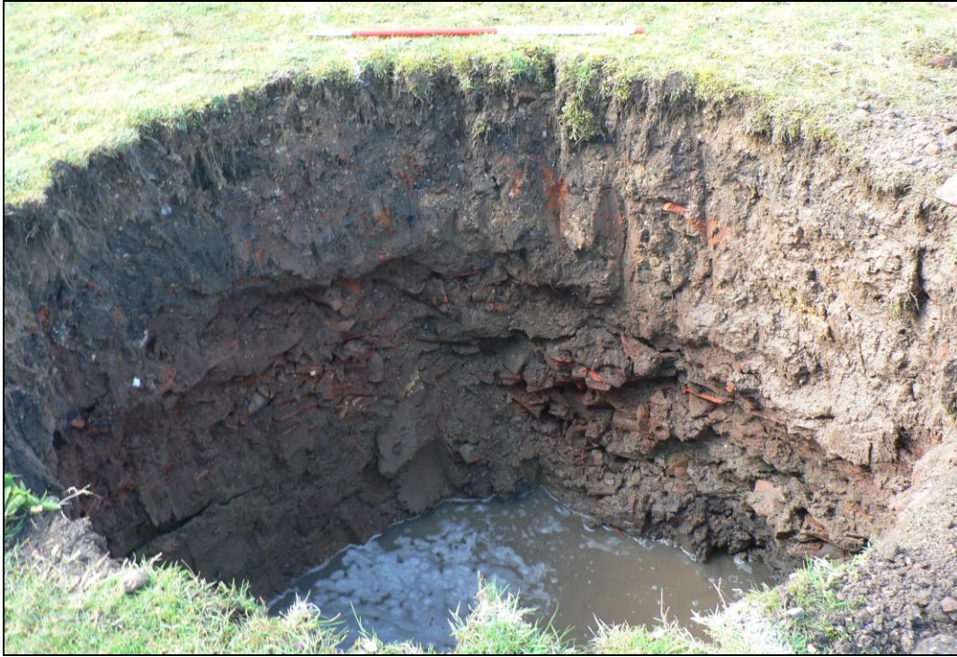
Treatment plant pit
