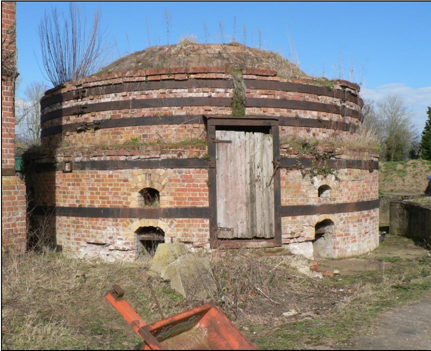
Kiln from northeast
