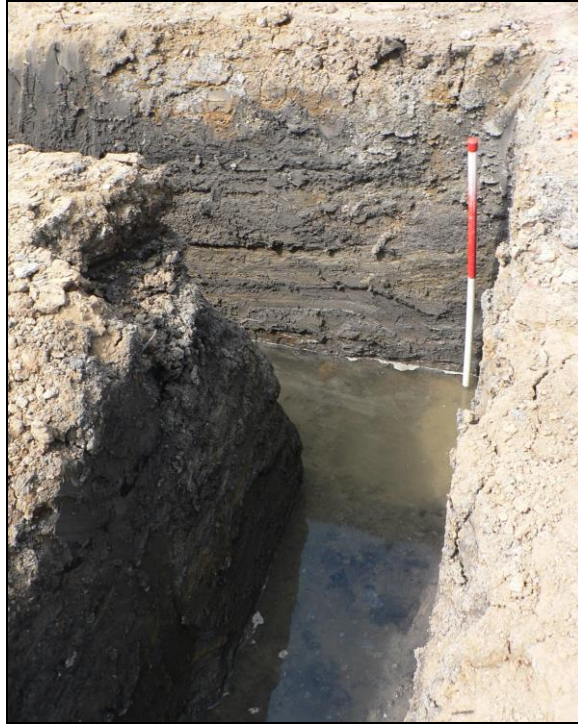
Southwest corner of foundations
