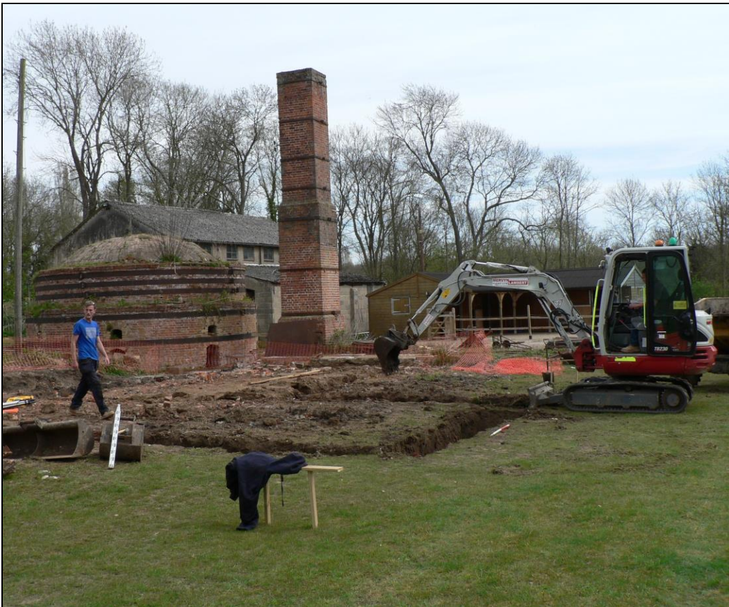
New build area from southwest following demolition of workshop
