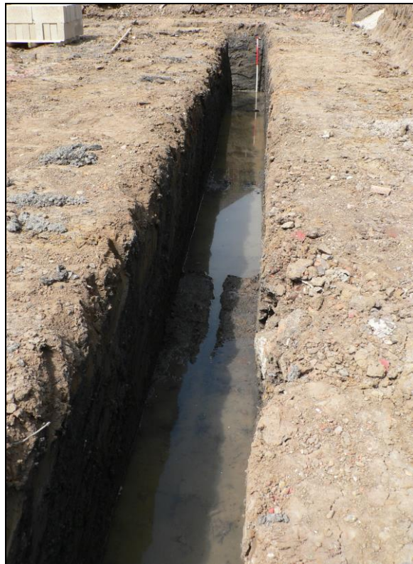
Northeast corner of foundations from west
