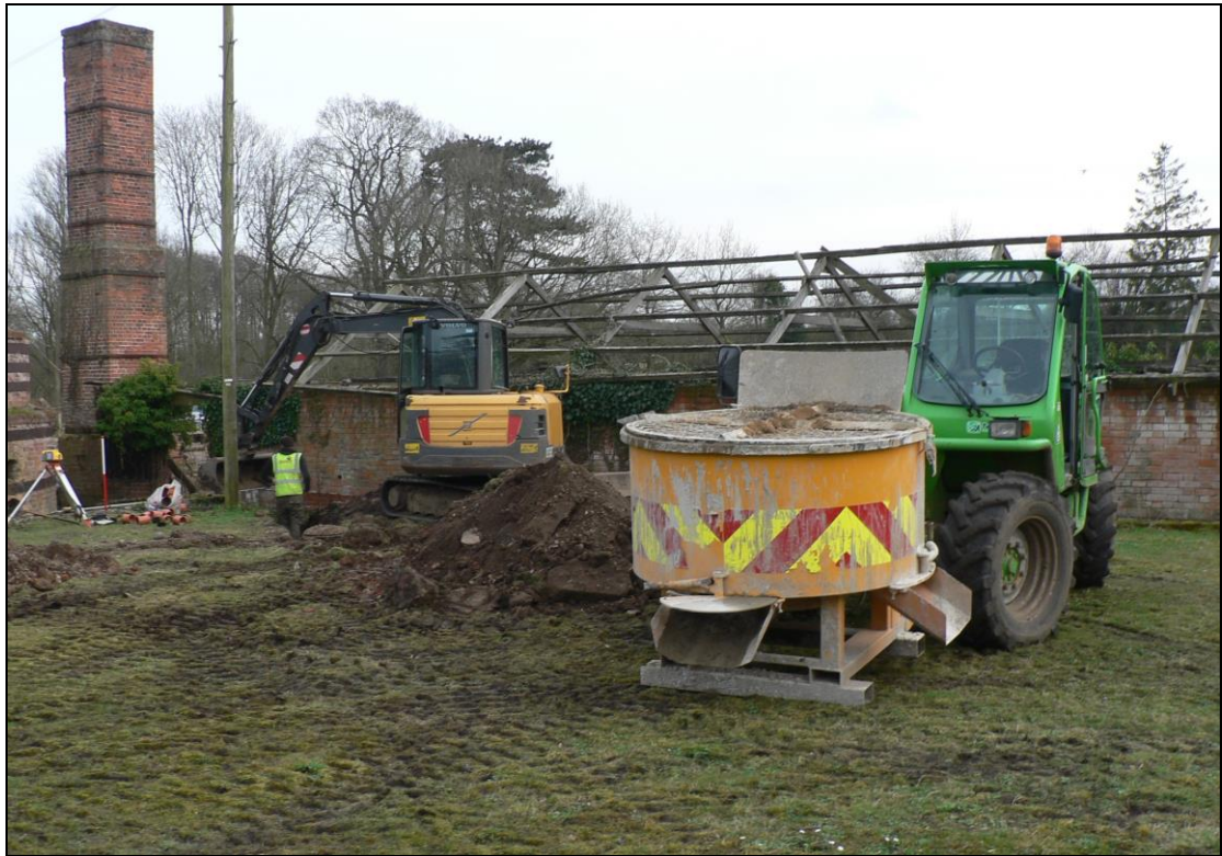
Treatment plant area from northeast
