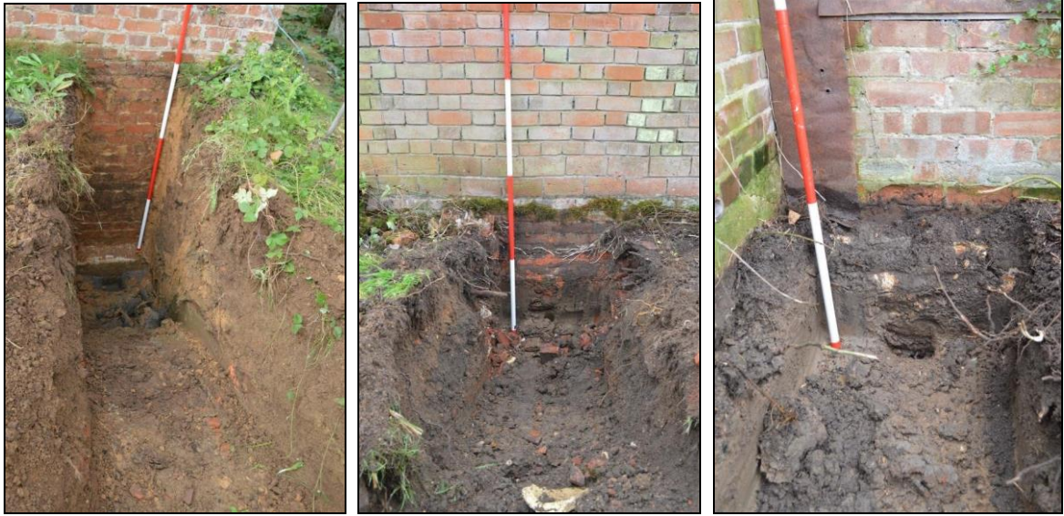
TP at eastern end of workshop TP on northern side of workshop TP at western end of workshop
