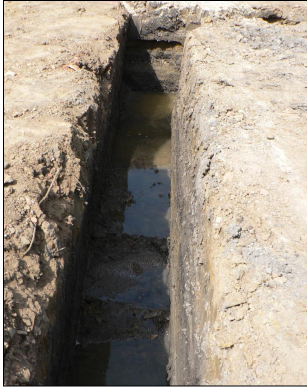
Eastern foundation trench
