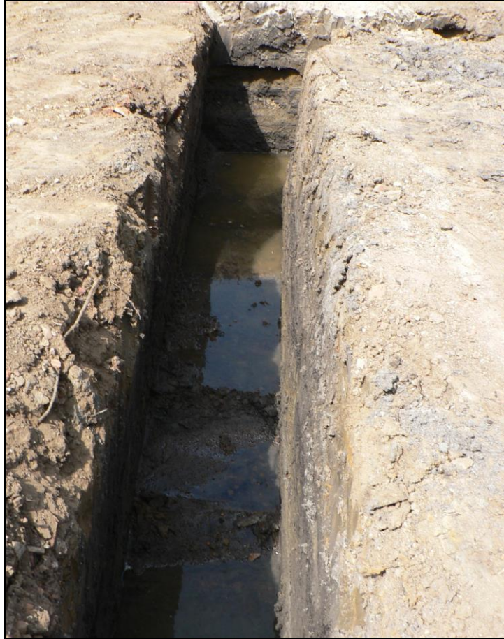
Western foundation trench
