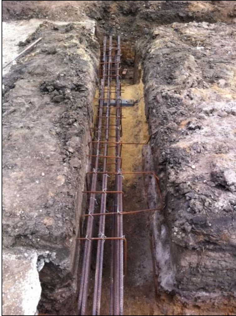
Oven 0006 towards top of image with sand & steel rods in place for foundation
