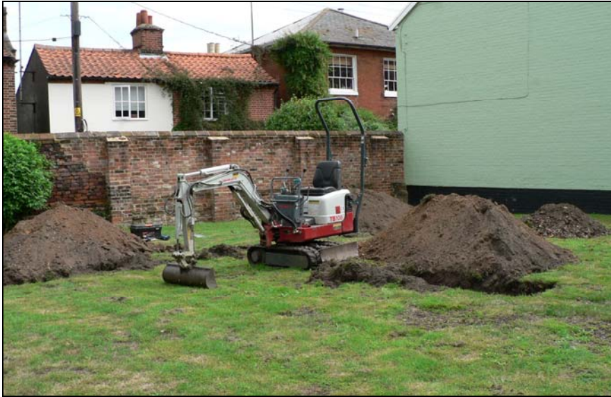
General view of evaluation area from north-west
