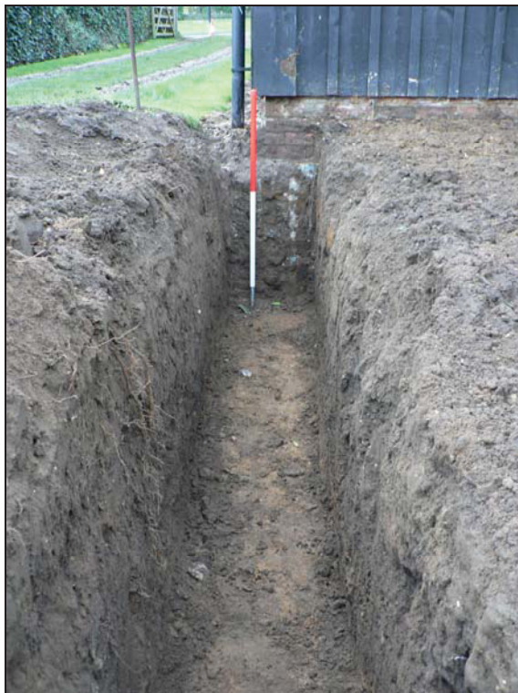
Southern foundation fully excavated from east
