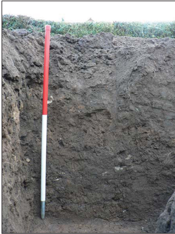
South east corner of foundations fully excavated
