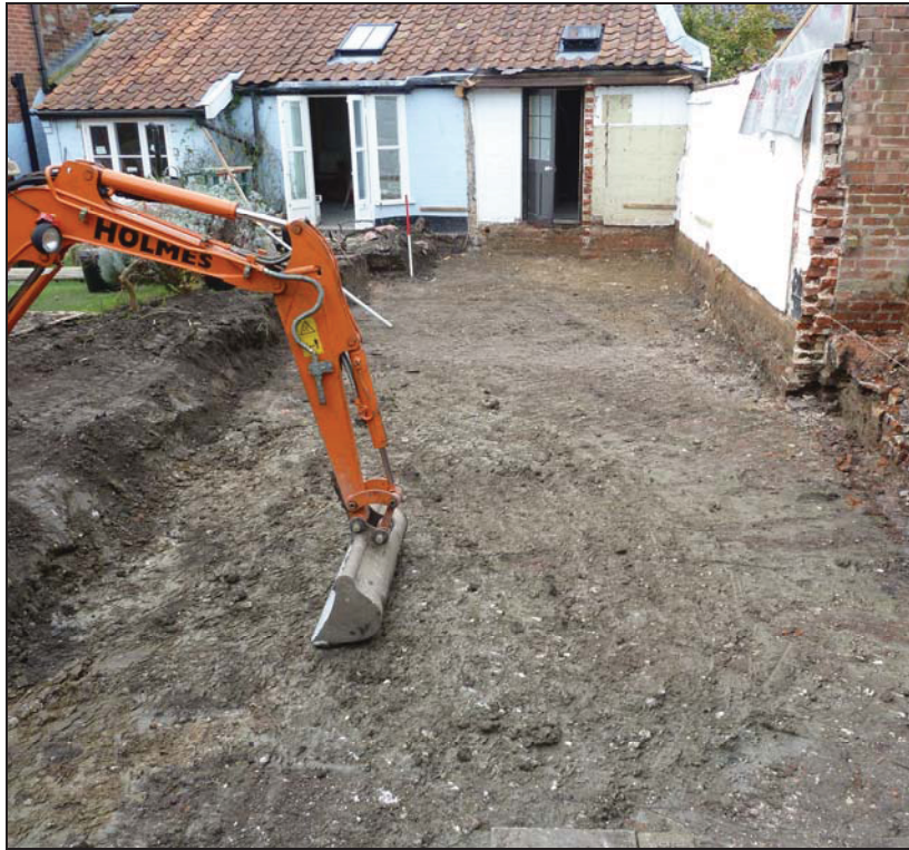
Stripped extension footprint from east
