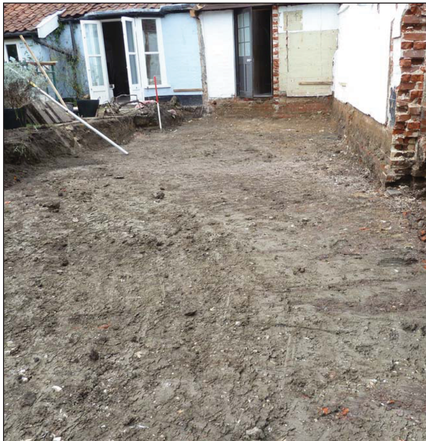
Stripped footprint from east- detail
