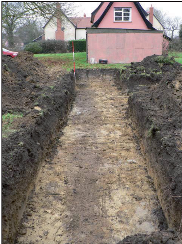
6. Main north-south aligned trench from south with ditch 0002 running along its length
