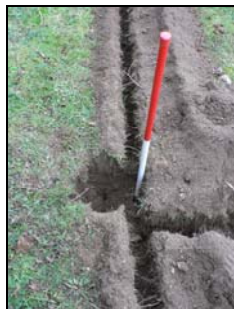
9. Narrow cable trench & post pit in paddock
