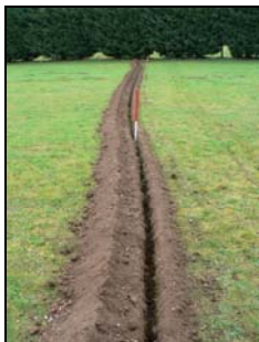
8. Narrow cable trench in paddock
