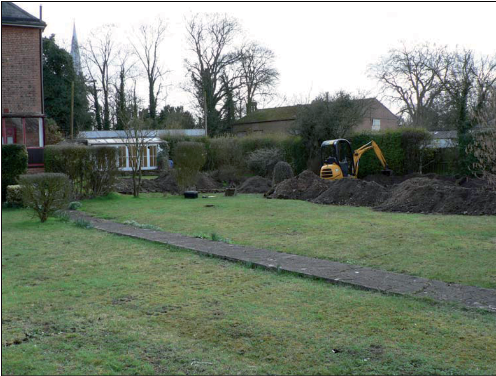
General view from north
