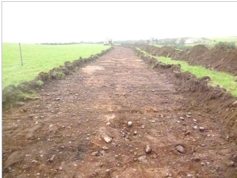
Figure 5b – post-ex of access track (middle section)
