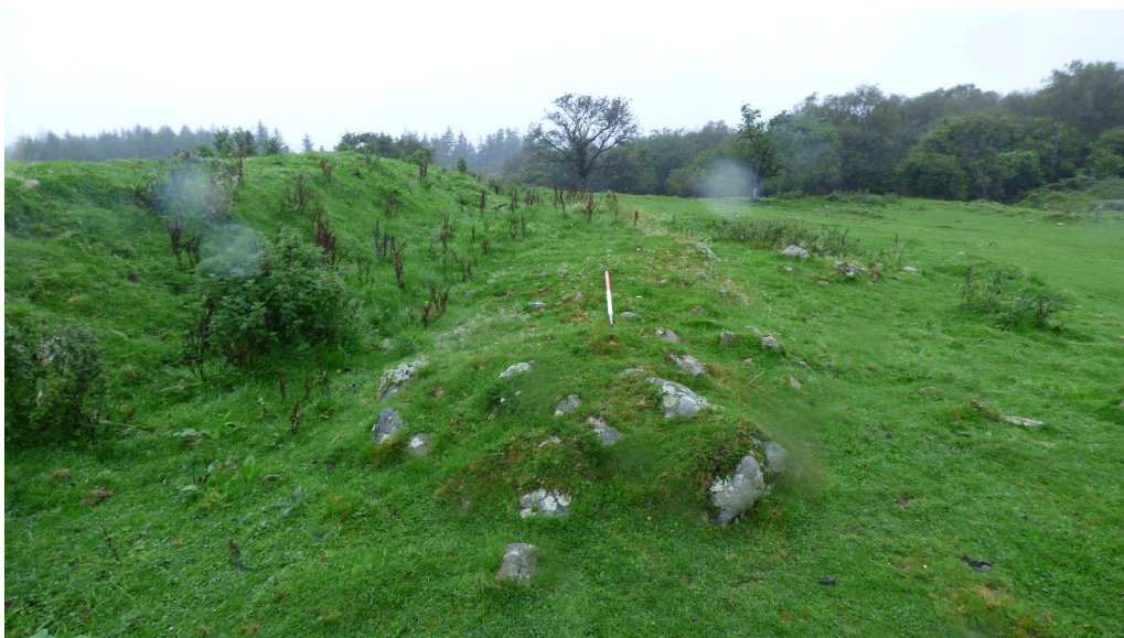
Figure 5c - section of walling close to exploratory pits (II) & (III) (from SE)
