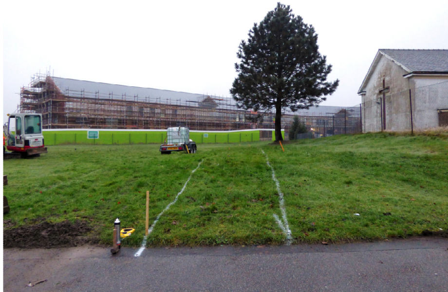
Figure 4a – pre-ex of trench 1 (from NE)
