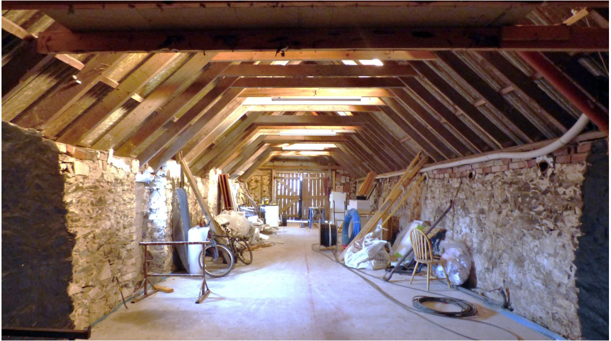
Figure 11a – general of single storey building (from SW)
