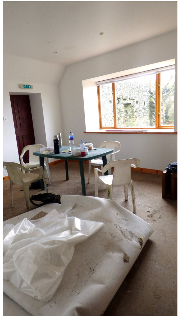
Figure 12c – general of upper floor of 2-storey building (office / tearoom)
