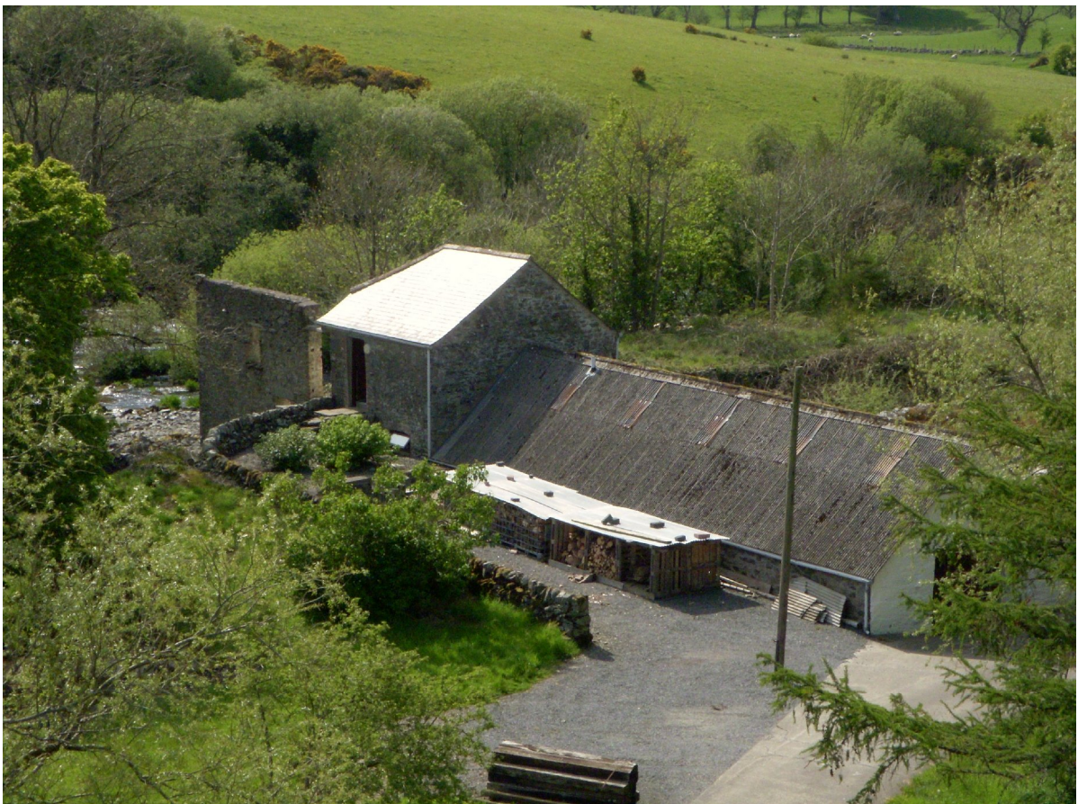
Figure 18b – aerial view of SE elevation of Torhouse Mill © Mark Davies (2012)
