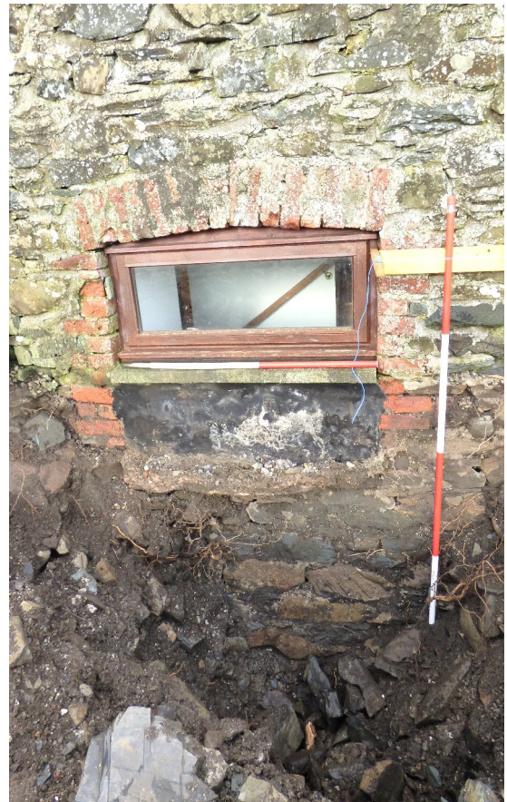
Figure 8c – partially blocked-in opening in SE elevation of 2-storey (from SE)
