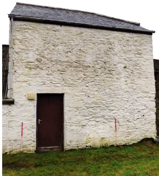
Figure 6b – NW elevation of 2-storey building showing entrance (from NNW)
