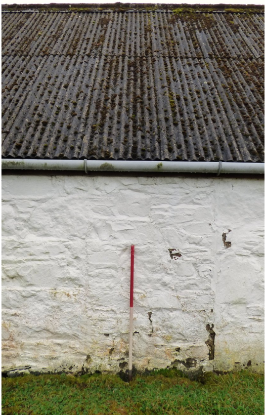
Figure 7c – infilled opening (III) in NW elevation of single storey (from NW)
