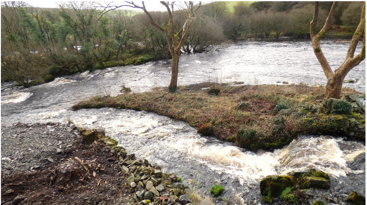
Figure 16b – showing where current lade / channel enters the river (tail race?) (from N)
