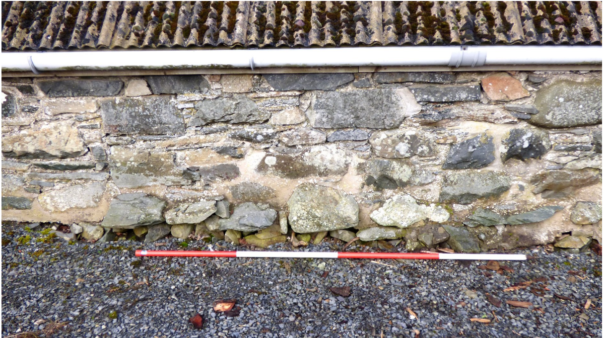
Figure 9a – showing stone protrusions in SE elevation of single storey building (from SE)
