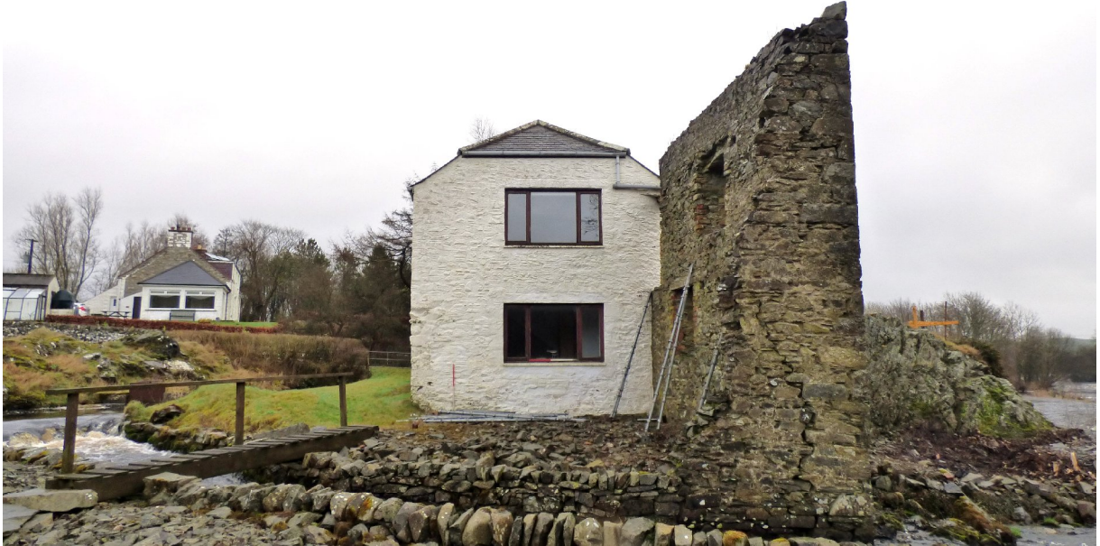
Figure 10a – SW elevation of 2-storey building & SE wall of ruinous building (from SW)
