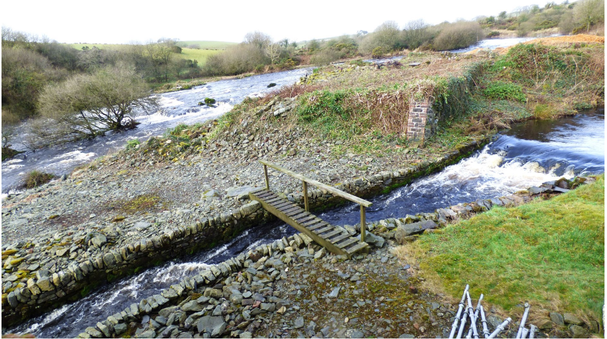
Figure 16a – looking WNW showing river, lade / channel and the demolished remains of the NW / SE range of mill buildings (from ESE)
