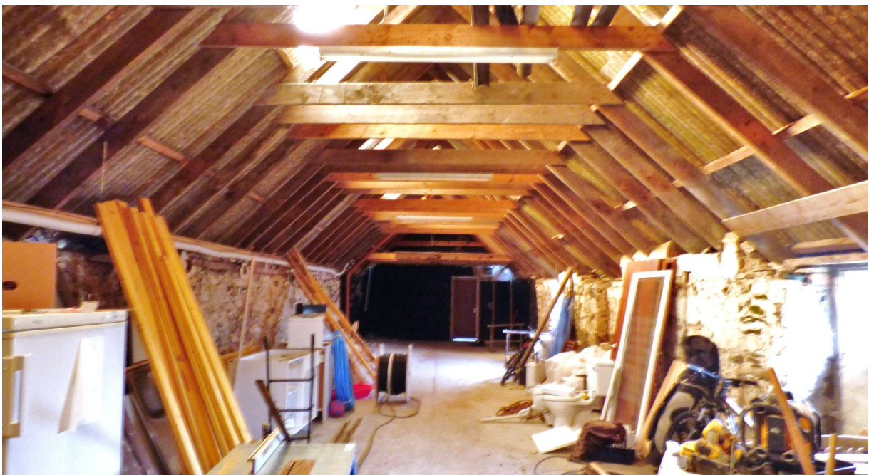
Figure 11b – general of single storey building (from NE)
