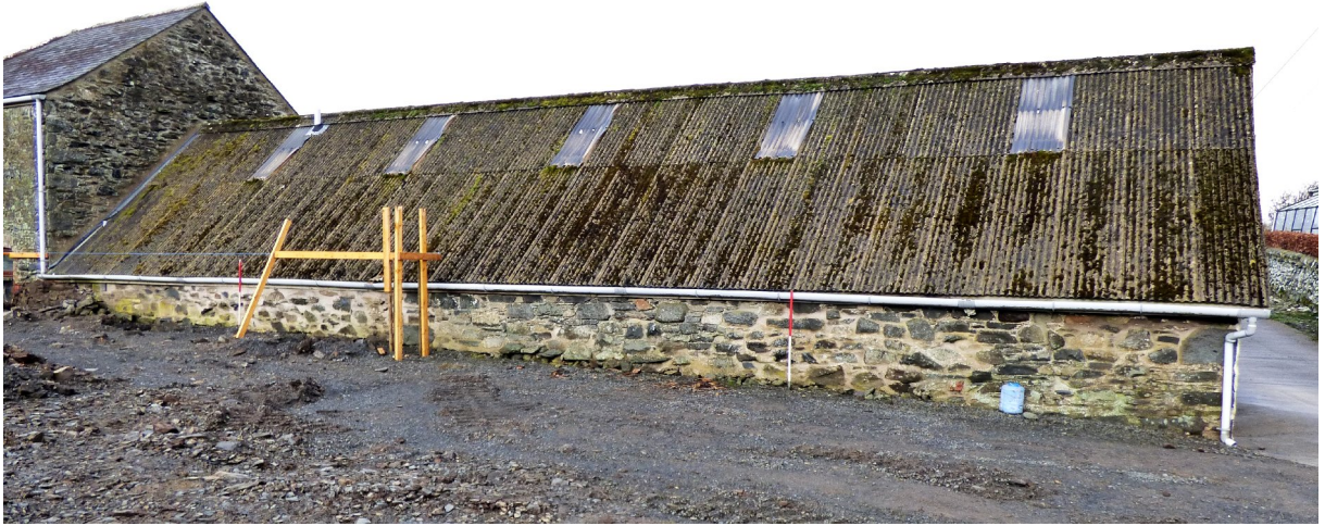
Figure 8a – SE elevation of single storey building (from ESE)
