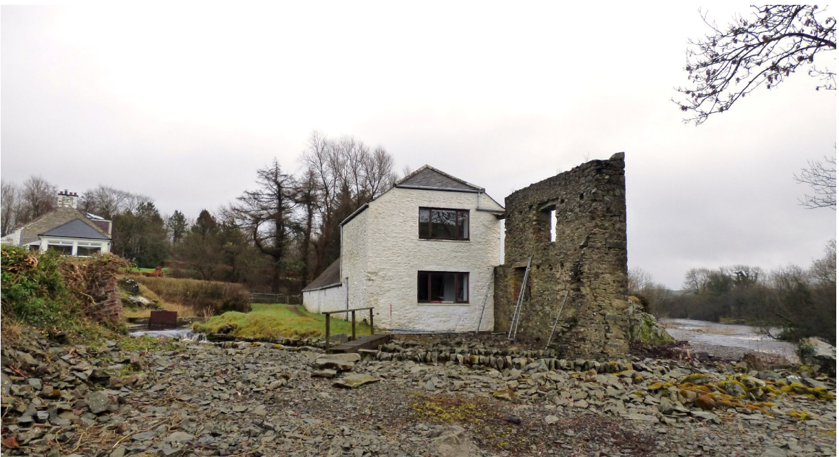
Figure 5c – general of existing mill buildings (from W)
