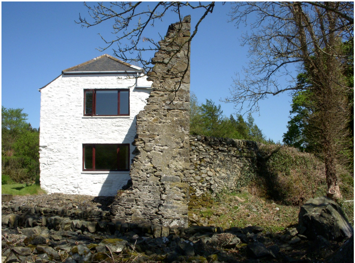
Figure 17b – ruinous 2-storey building; SW elevation of 2-storey building & revetment wall (from SW) © Mark Davies (2012)
