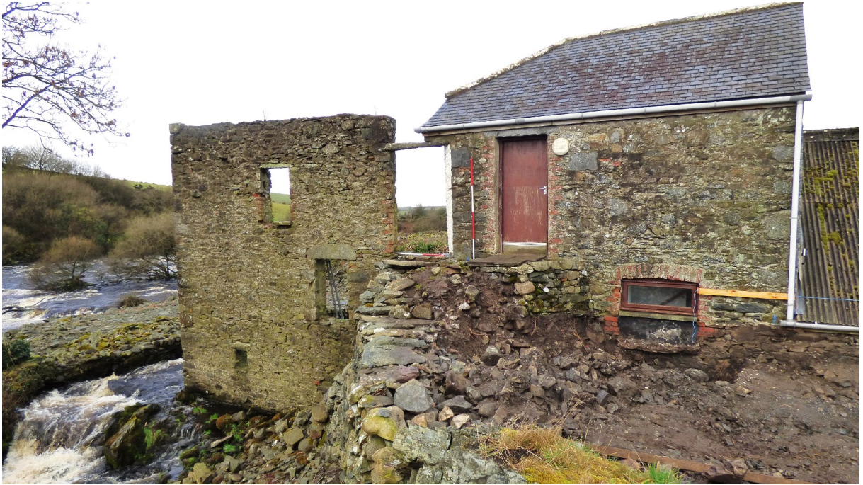
Figure 14a – SE elevation of 2-storey building & 2-storey ruinous building (from ESE)
