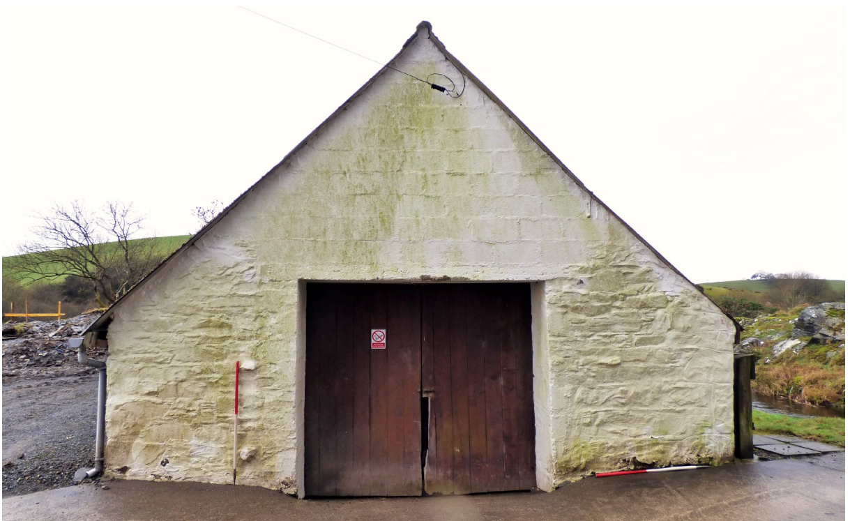
Figure 10b – NE gable of single storey building (from NE)
