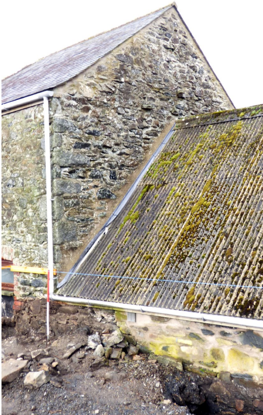
Figure 8b – SW gable of 2-storey building (from ESE)
