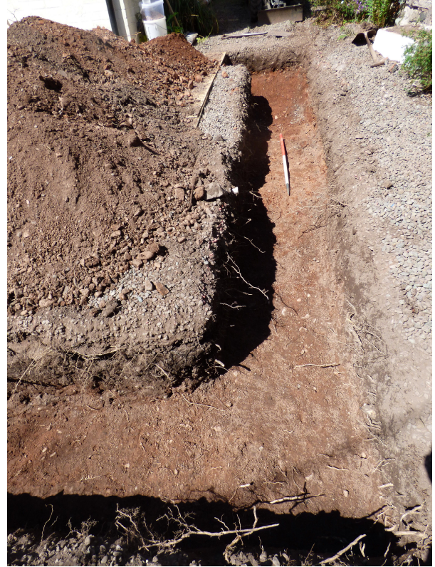
Figure 7b - post-ex of foundation trench B (From E)
