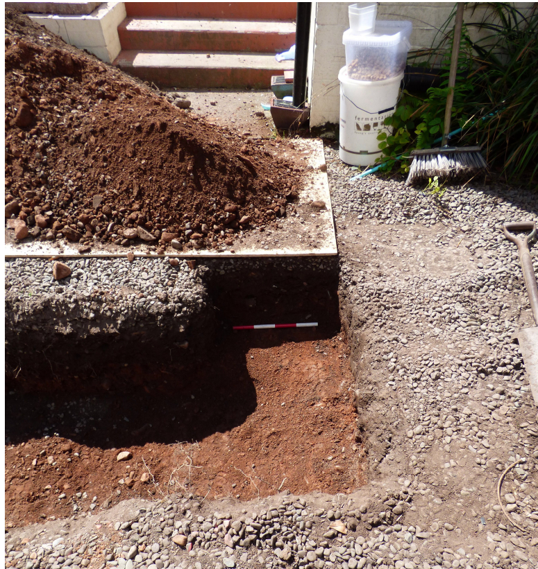
Figure 8a - post-ex of foundation trench C (from N)
