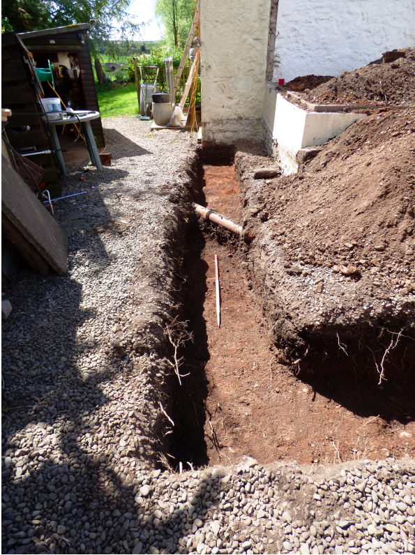
Figure 7a - post-ex of foundation trench A (from N)
