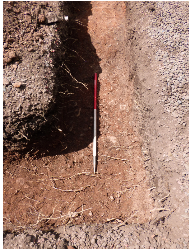
Figure 7d - northeast corner of foundation trenches (From E)
