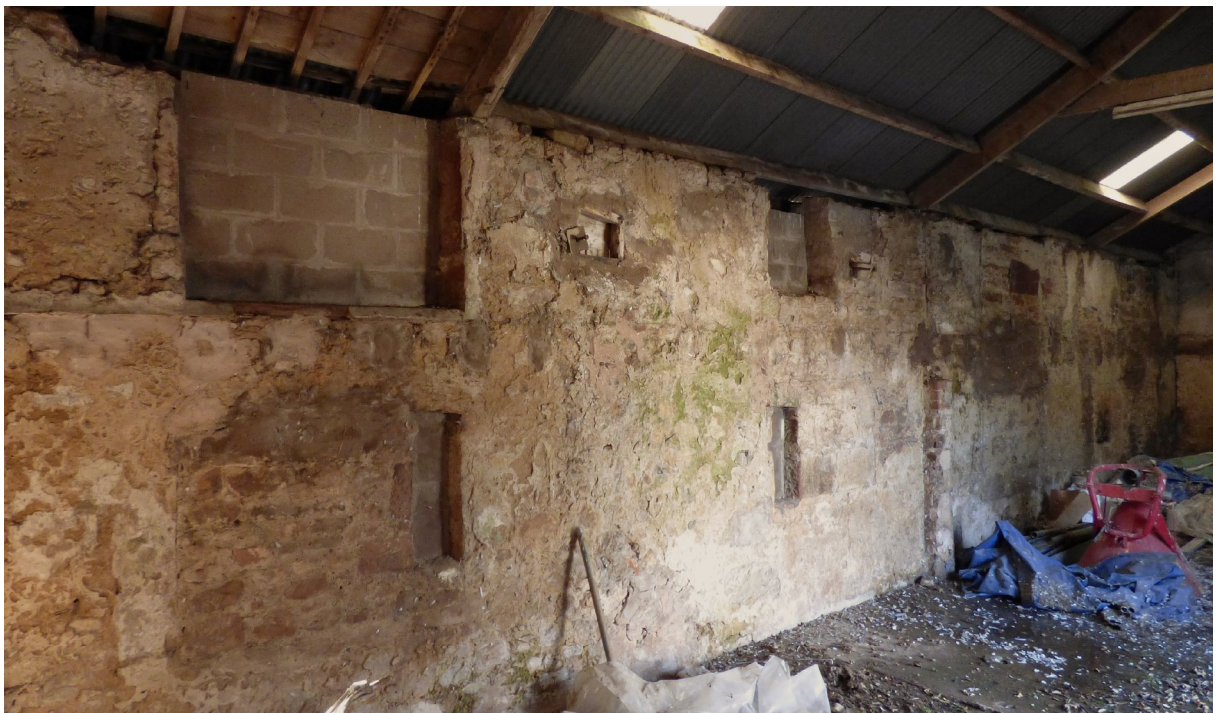
Figure 15c – detail of infilled openings within SE elevation - south-eastern range (from ESE)
