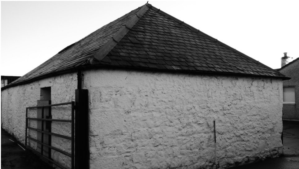
Figure 4b – SW (end) wall - north-western range (from WNW)
