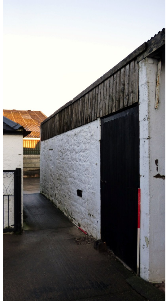
Figure 18b – SW elevation (NW half) - north-eastern range (from SSE)
