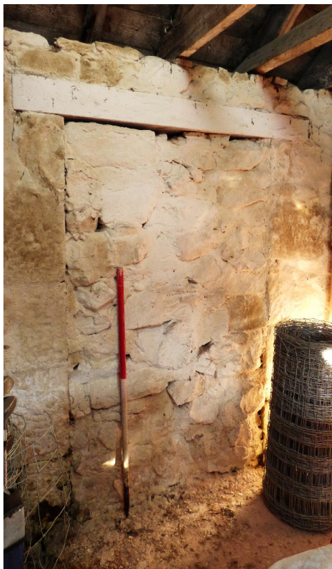
Figure 5c – blocked-in doorway in NW elevation - SW range (from SSE)
