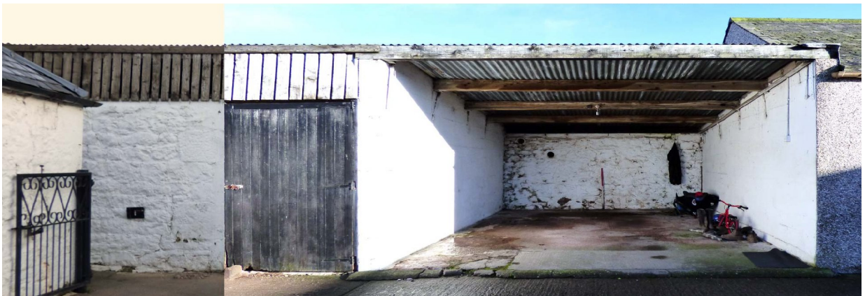
Figure 8b – SW elevation of NW half - north-eastern range (from SW)
