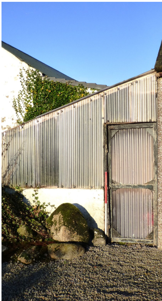
Figure 16b – 'greenhouse' attached to SW end – SE range (from SE)
