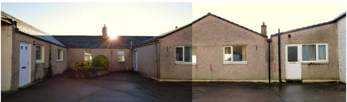
Figure 17c – NW elevation - south-eastern range (dwelling) (from NW)
