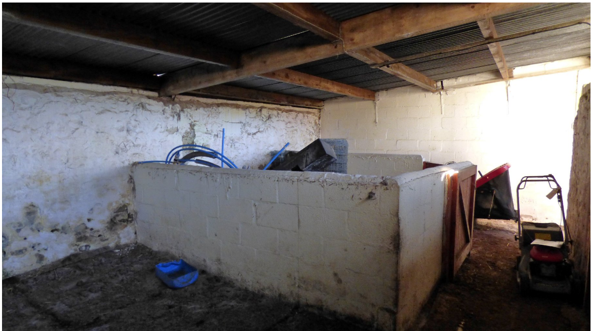
Figure 18c – general view of interior - north-eastern range (from W)
