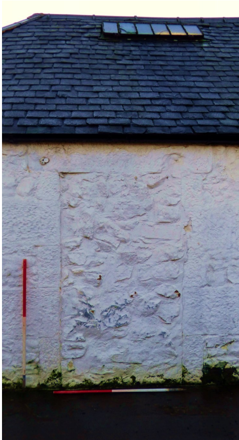
Figure 5a – blocked-in doorway in NW elevation - SW range (from NW)
