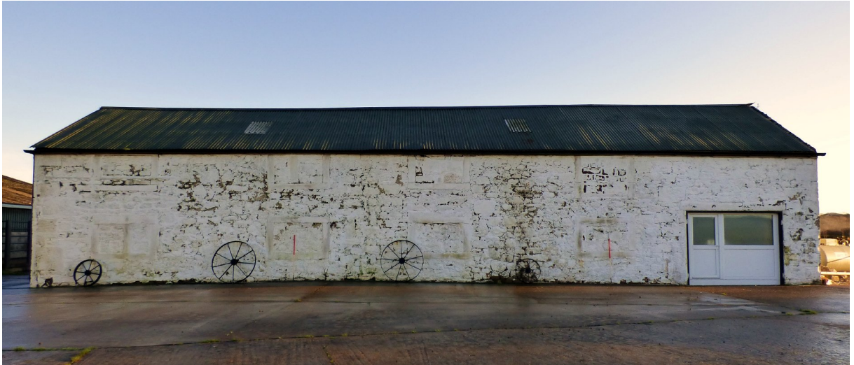
Figure 10a – SE elevation - south-western range (from SW)
