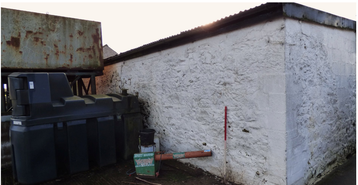
Figure 8c – part of NE elevation (NW half) - north-eastern range (from N)
