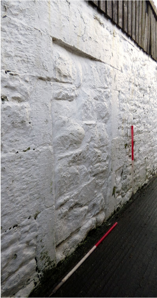
Figure 9a – blocked-in doorway in SW Elevation - NE range (from WSW)
