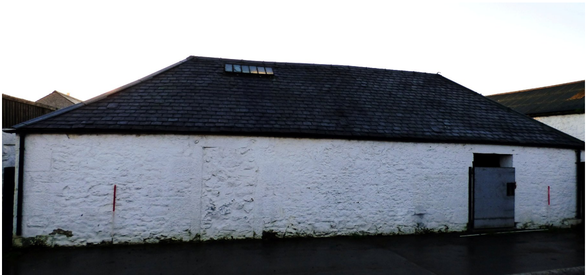
Figure 4c – NW (rear) elevation - north-western range (from NNW)
