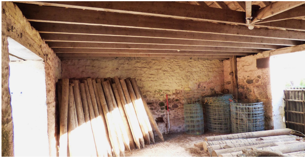
Figure 6b – gable (in middle) - north-western range (from W)
