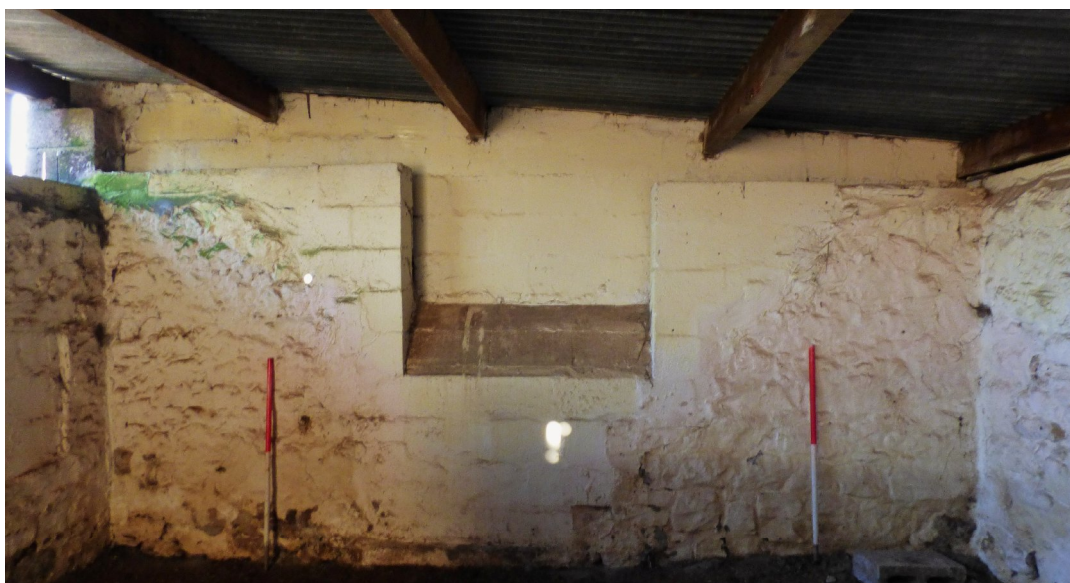
Figure 7c – showing later blockwork at NW (end) wall - north-eastern range (from SE)
