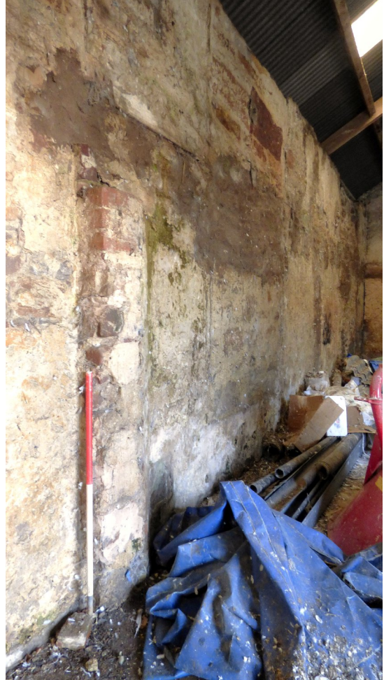
Figure 15b – narrow 'buttress' protruding from SE elevation – SE range (from ESE)
