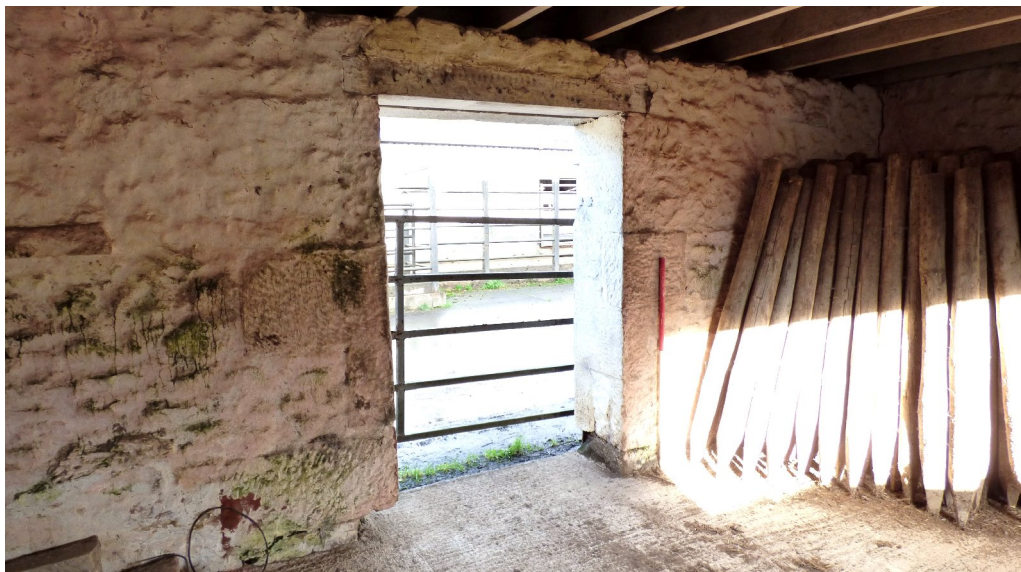
Figure 6c – entrance at SW end of NW elevation - north-western range (from S)
