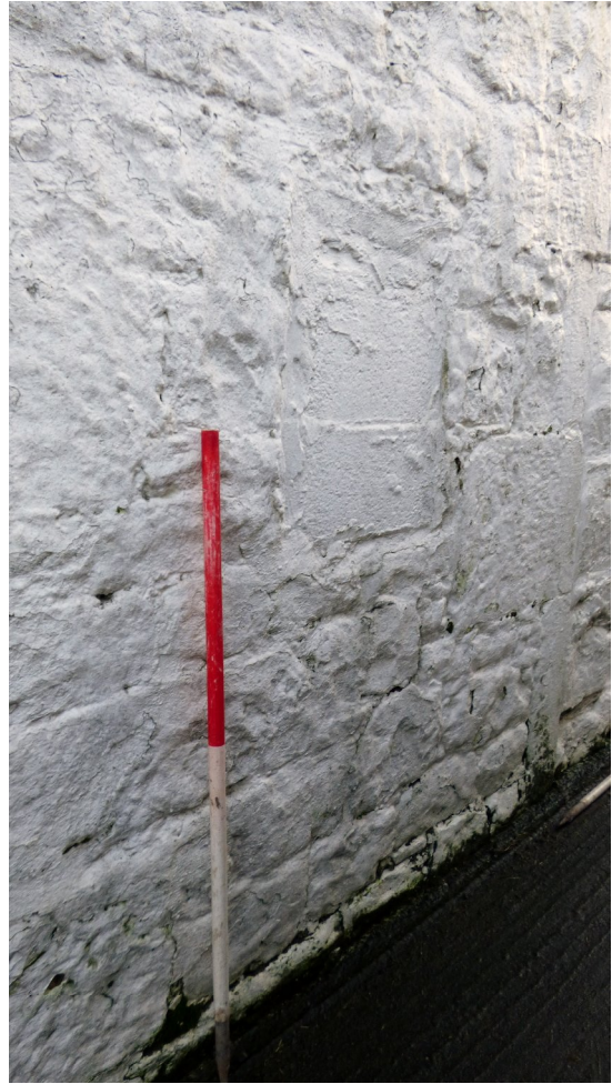
Figure 9b – blocked-in window in SW elevation - NE range (from WSW)
